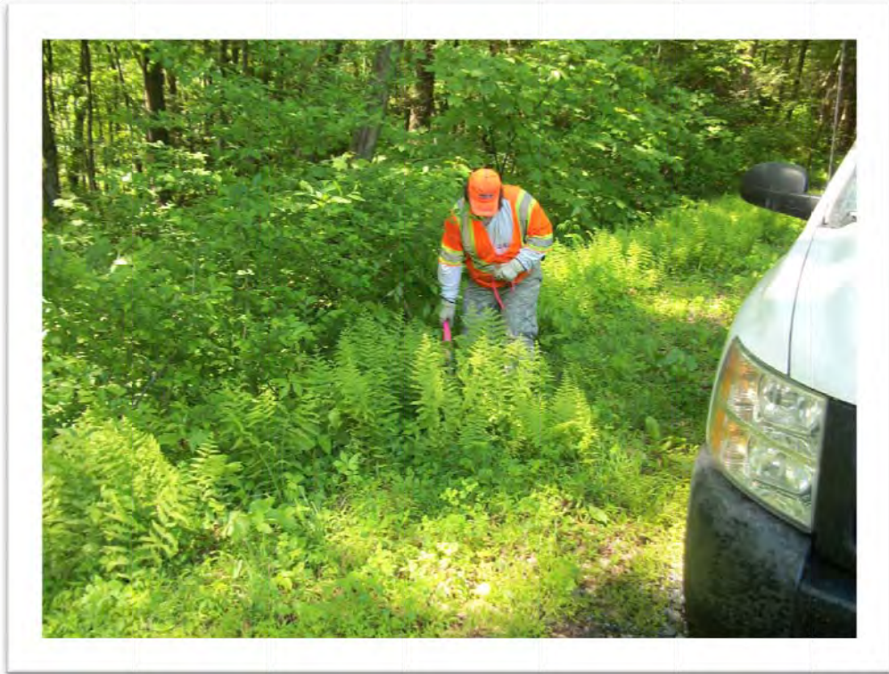
Technician removing survey stakes and flagging tape in SGL211
