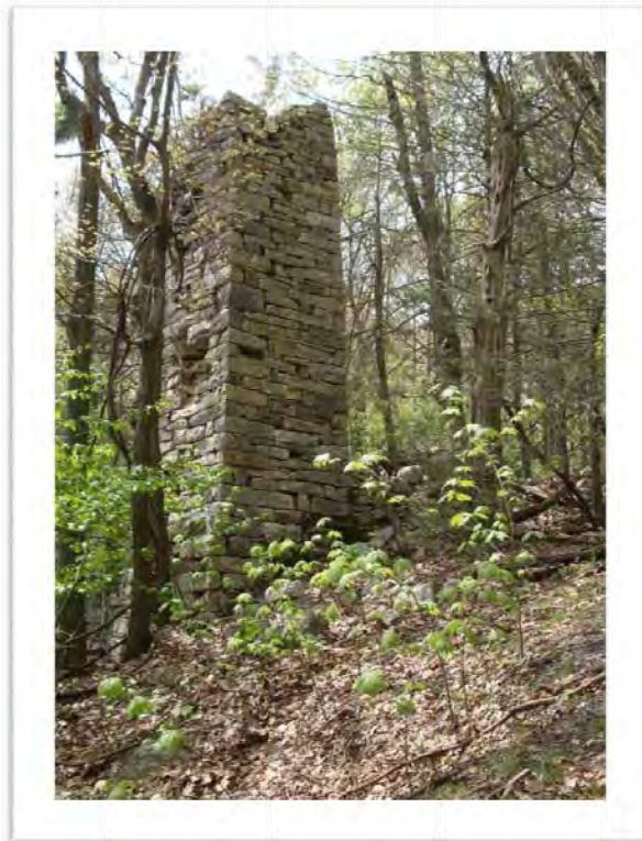
Stone smokestack structure on VS-26.
