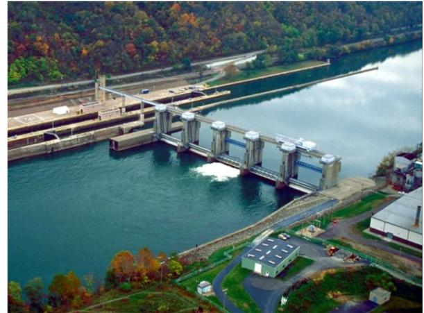
**Figure 7.2.** Monongahela River L/D 4 at Charleroi (RM 41.5). Even with only the middle tainter gate open, water velocity downstream of the dam is appreciably higher than upstream (from USACE 2010).
