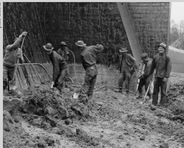
Members of a CCC crew work on the foundation of the dam that created Laurel Hill Lake at Laurel Hill State Park.
