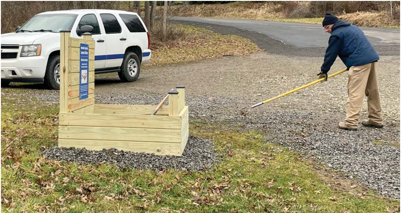
An AIS composting station being installed at Tamarack Lake, Crawford County.
