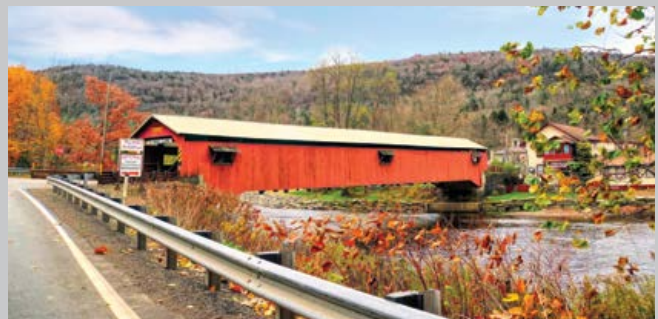
Forksville Covered Bridge, Sullivan County
