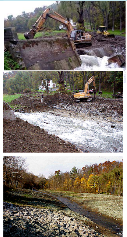
Removal of Reedsville Dam on Tea Creek (Mifflin County)
