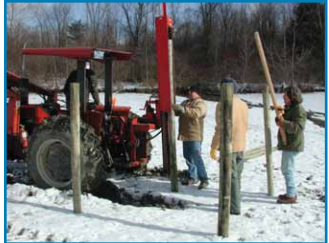
Pennsylvania post cluster construction
