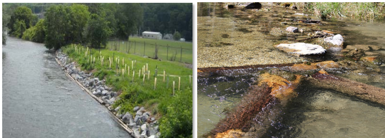
Figure 24. Riparian buffer and streambank stabilization project along Spring Creek, Centre County (left) and instream trout habitat improvement project in Big Spring Creek, Cumberland County (right).
