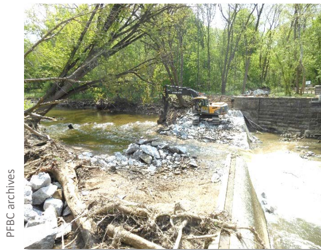
Figure 23. Heistand Sawmill Dam removal.
