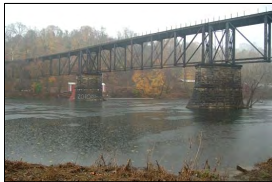
Eastern and Northern EA - 77A Bridge (near 9 th Street)
