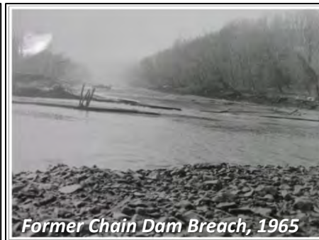
Former Chain Dam Breach, 1965
