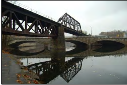
Dr. George S. Smith Bridge (3 rd Street / S.R. 611) (Concrete Arch Bridge)
