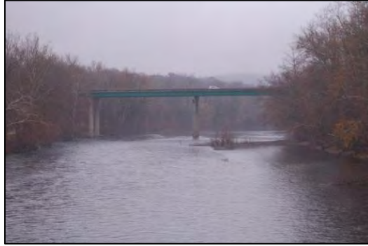
Glendon-Wilson Bridge (25 th Street / S.R. 2012)
