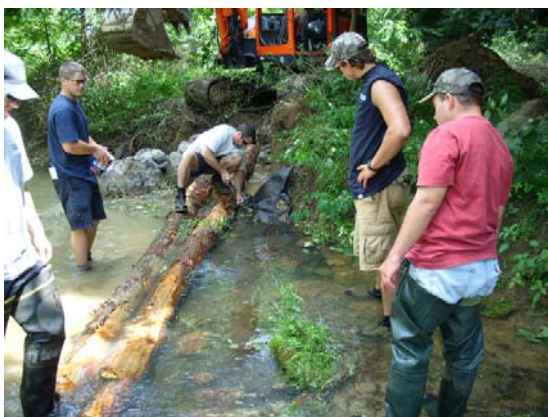
Installing habitat improvement structure. Photo: Northcentral PA Conservancy
