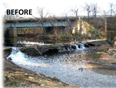
Old Huntingdon Pike dam removal, Pennypack Creek
