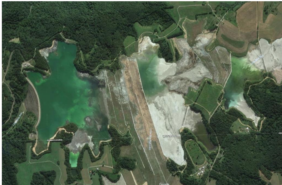
Figure 4.3.21-3 Little Blue Run Coal Ash Pond along the Pennsylvania-West Virginia Border (Frazier, 2018a)
