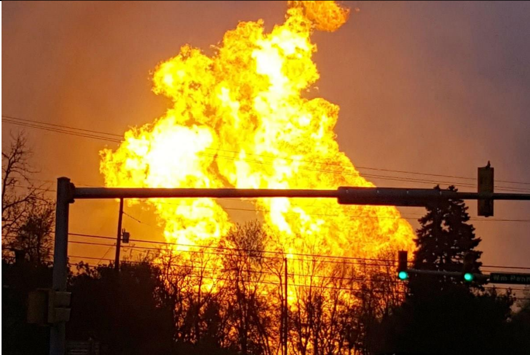
Figure 4.3.23-3 Photograph of an explosion on a 30-inch interstate natural gas pipeline in rural Salem Township, Pennsylvania. Source: NPR State Impact.
