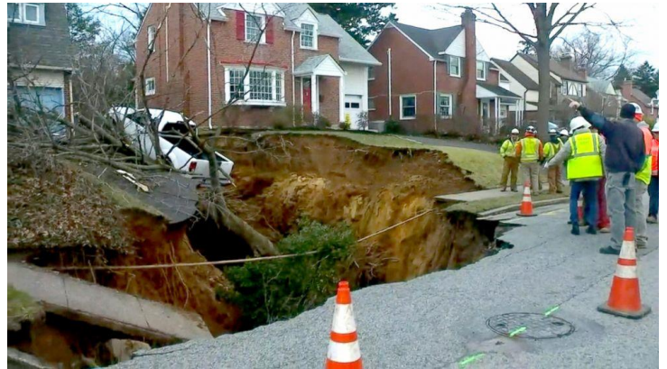
Sinkhole in Philadelphia in private home's front yard (Tan, 2017).
