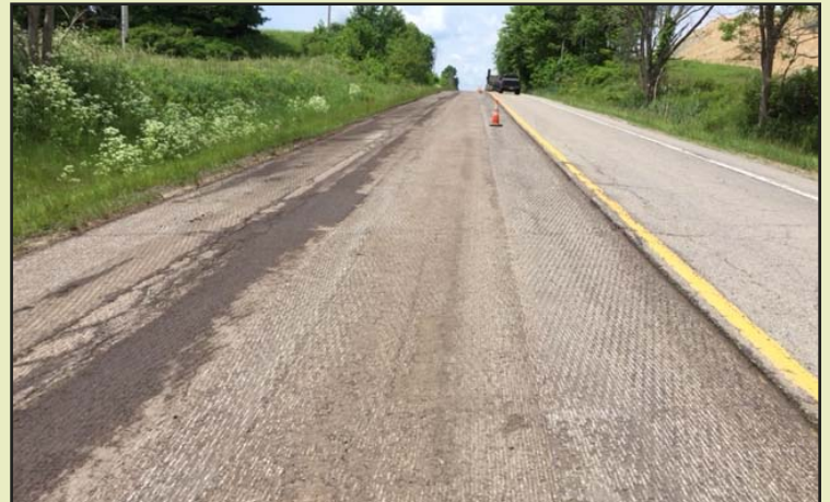
One lane of this roadway has been milled away in preparation for the placement of Recycled Asphalt Pavement.
