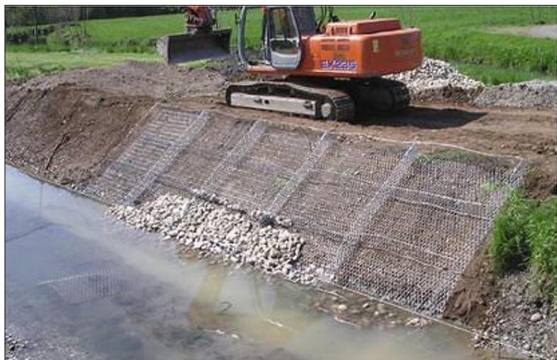
Figure 10-37 - Reno Mattress Installation [55]
