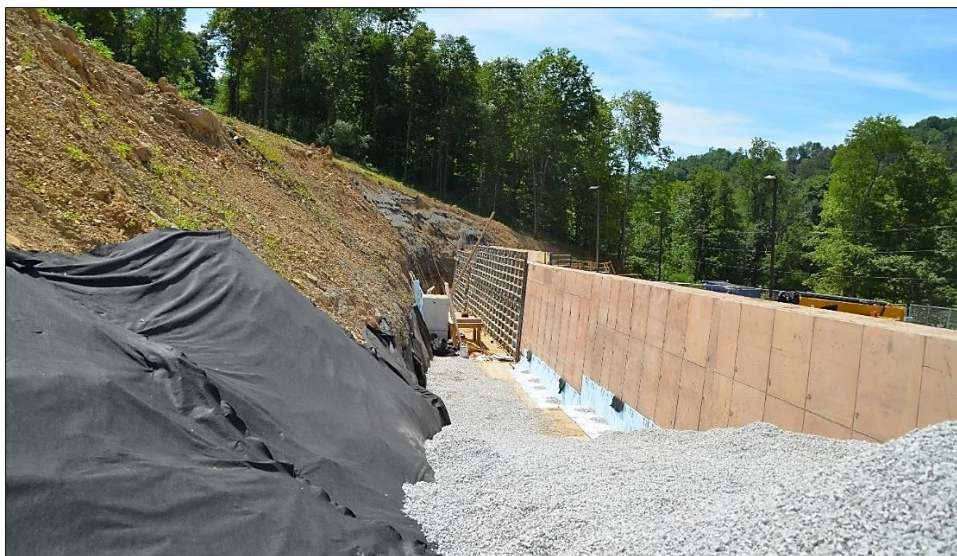
Figure 10-43 - Concrete Gravity Wall Construction, Landslide Repair
