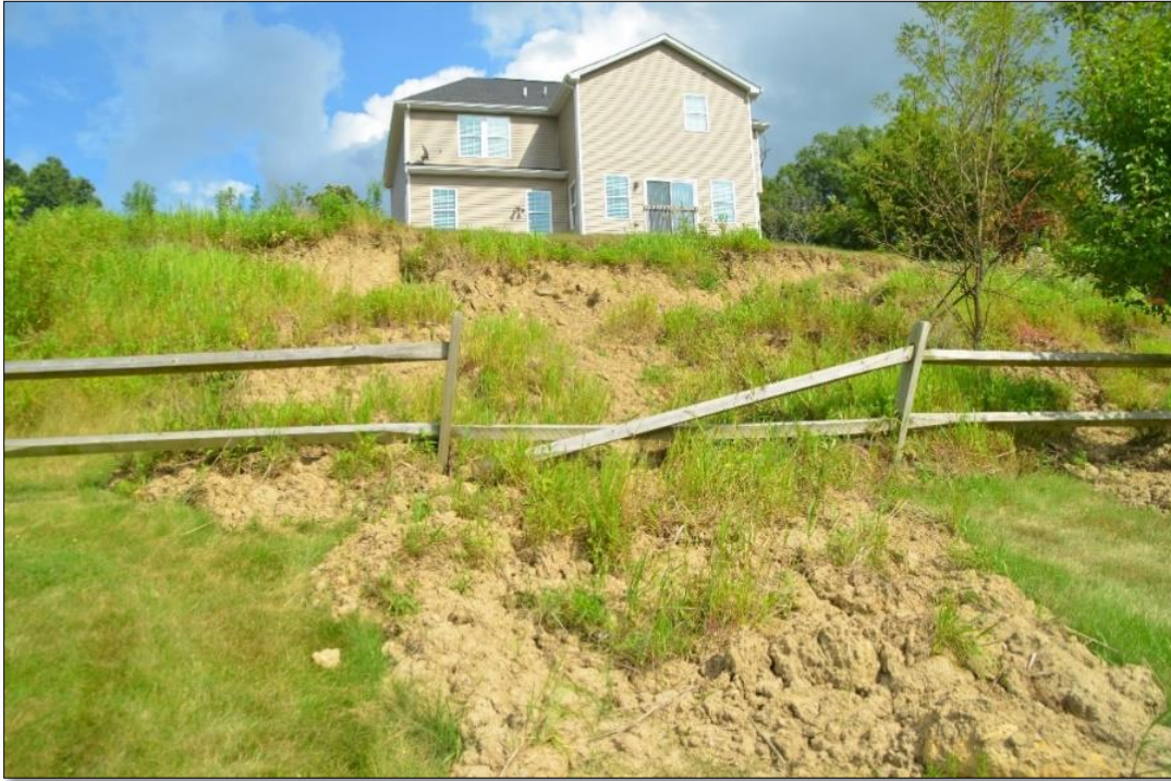
Figure 10-109 - Existing Rotational Slide
