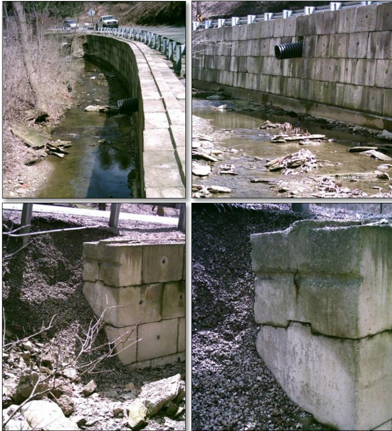
Figure 10-49 - Modular ("Jumbo") Block Wall
