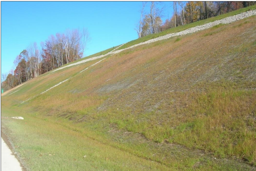
Figure 10-99 - Finger Drains on Slope
