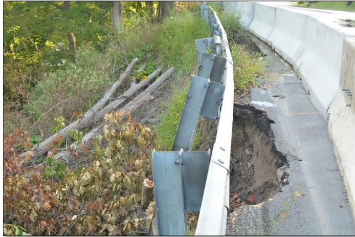
Figure 10-55 - Landslide at edge of shoulder
