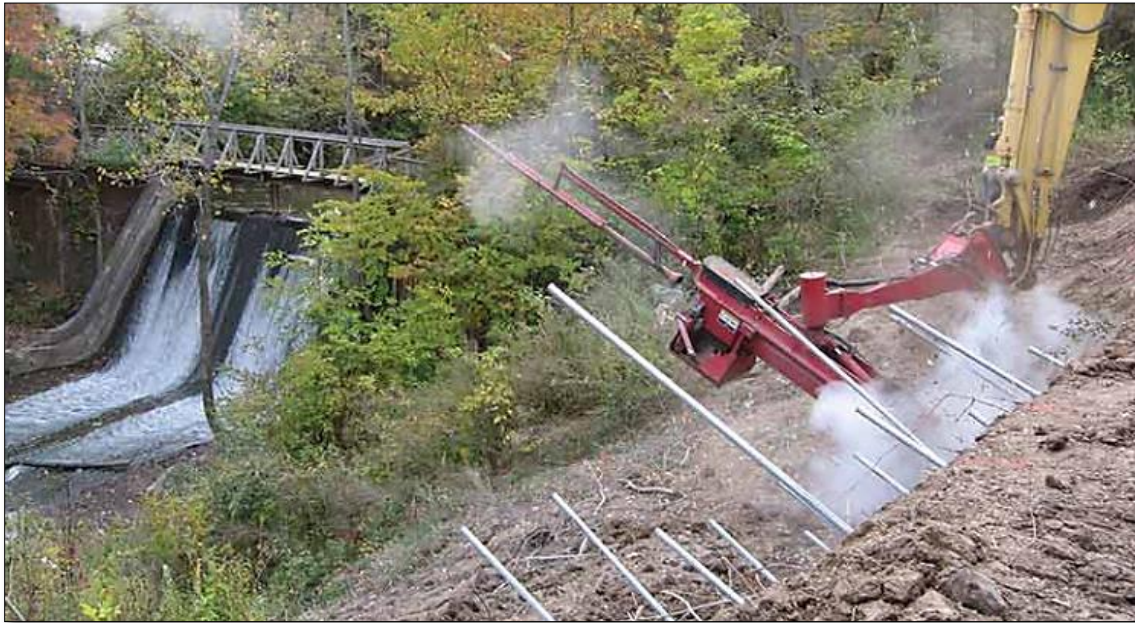
Figure 10-81 - Soil Nail Launcher [13]
