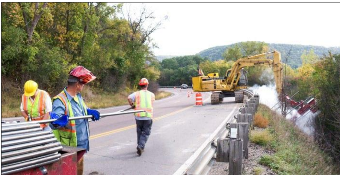
Figure 10-82 - Soil Nail Launcher [57]
