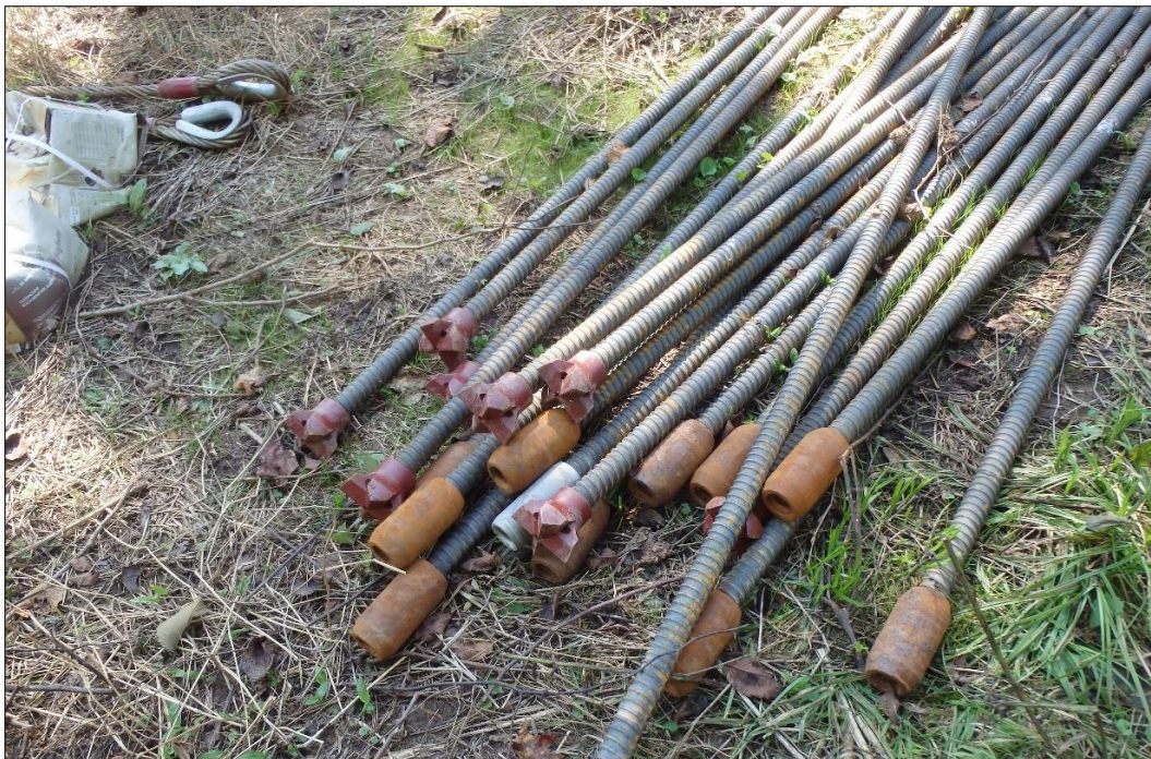
Figure 10-74 - Soil Nails
