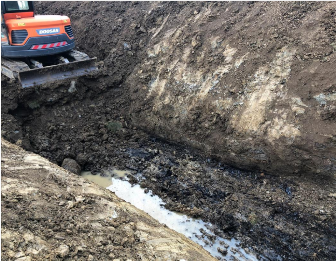
Figure 10-110 - Toe Key Excavation
