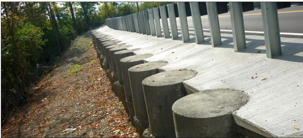
Figure 10-59 - Tangent Pile Wall Supporting Roadway Shoulder [23]
