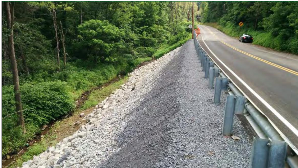
Figure 10-39 - Shoulder Back-Up
