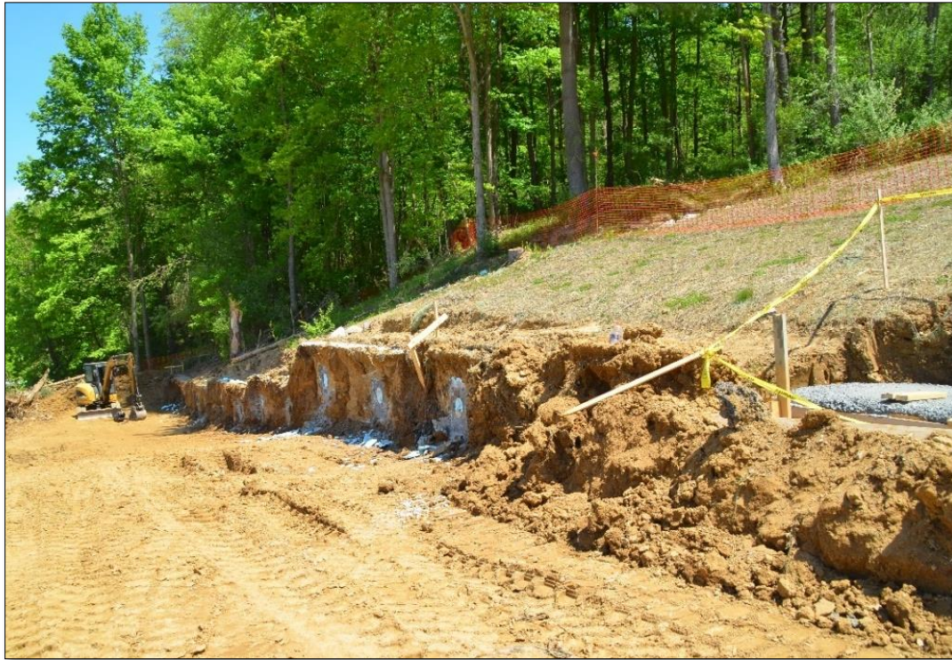
Figure 10-69 - Example Buried Panel Wall with Tiebacks, Front Face of Panel Partially Exposed
