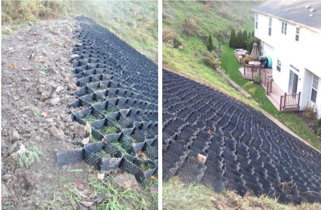
Figure 10-23 - Geocell Installation
