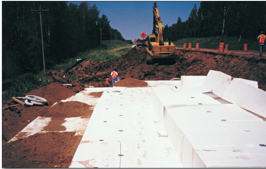
Figure 10-105 - Geofoam for Landslide Repair [124]
