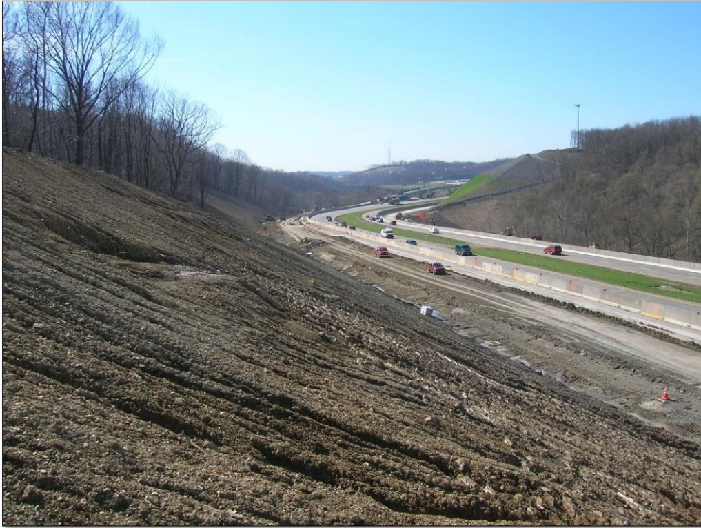
Figure 10-98 - Slope cleared to allow for identification of seepage points and installation of finger drains
