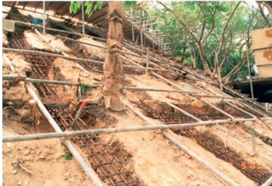
(a) Construction of soil nails and grillage.
