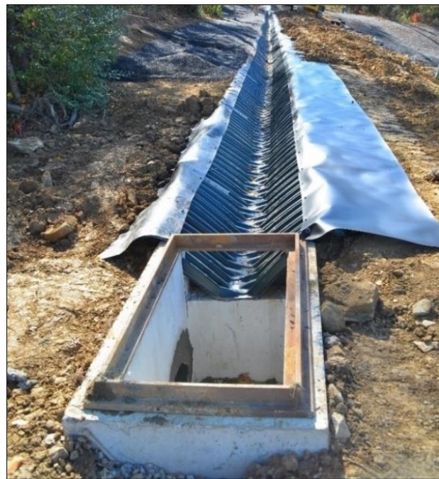
Figure 10-88 - Smart Ditch
