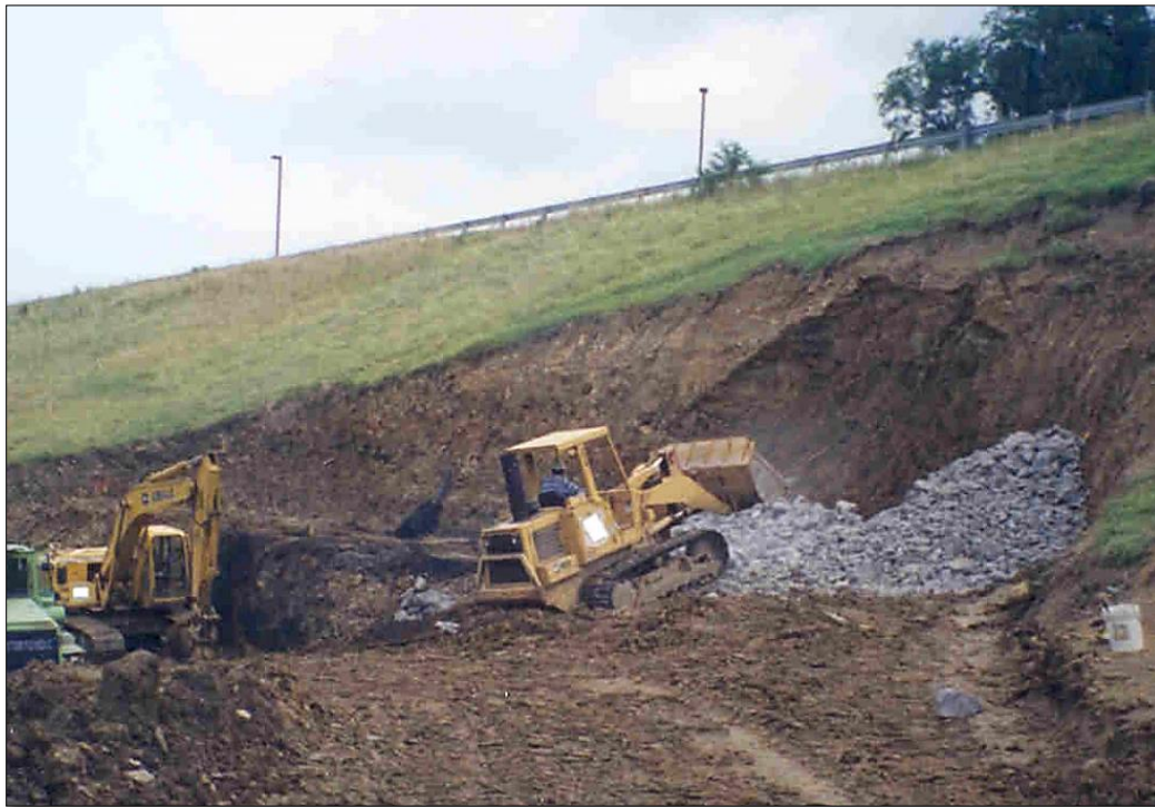
Figure 10-13 - Construction of Rock-Fill Buttress to Repair Landslide
