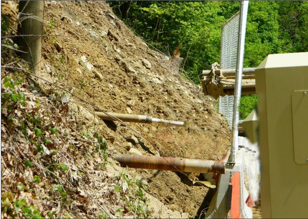
Figure 10-103 - Slotted Well Screen and PVC Conveyance Pipe Through Surface Casing to Install Horizontal Drains
