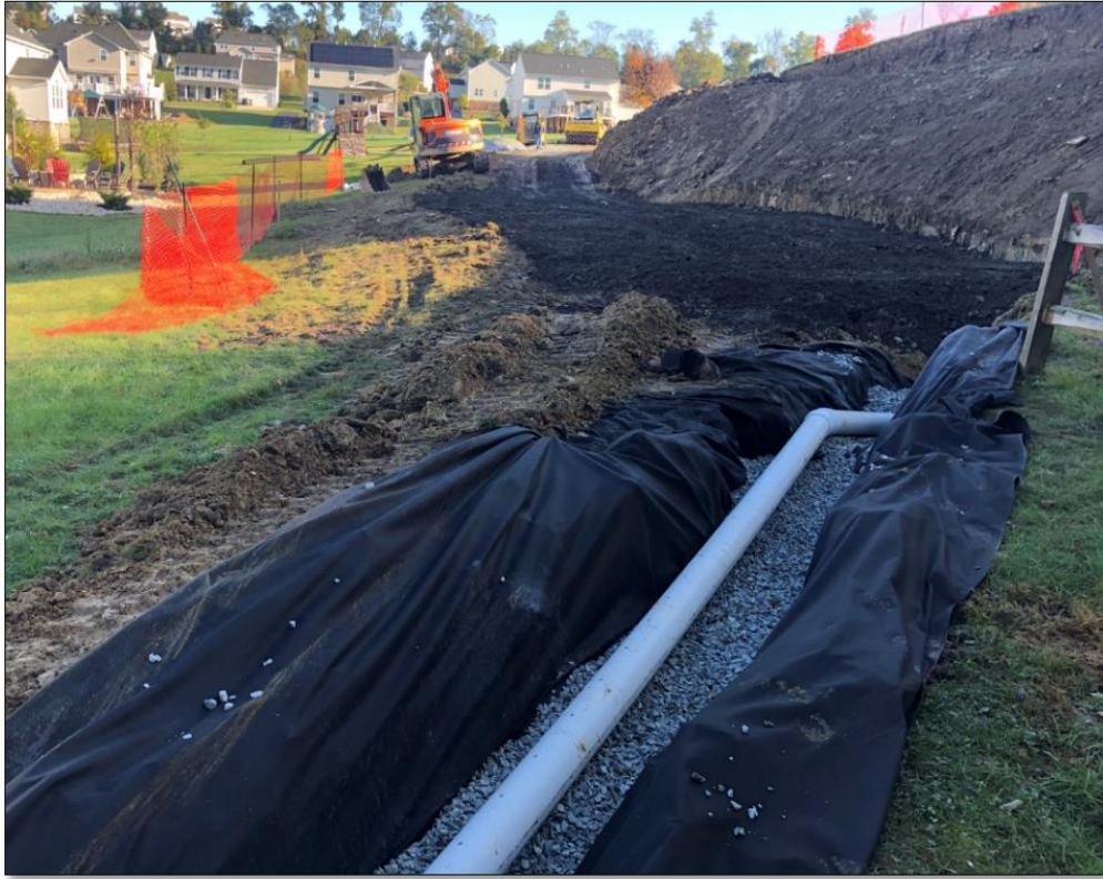
Figure 10-111 - Drain Installation in Toe Key
