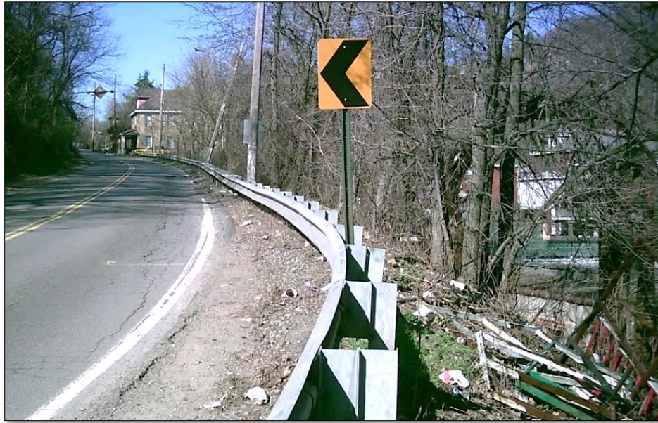
Figure 10-50 - Distressed Roadway Before Slope Repair
