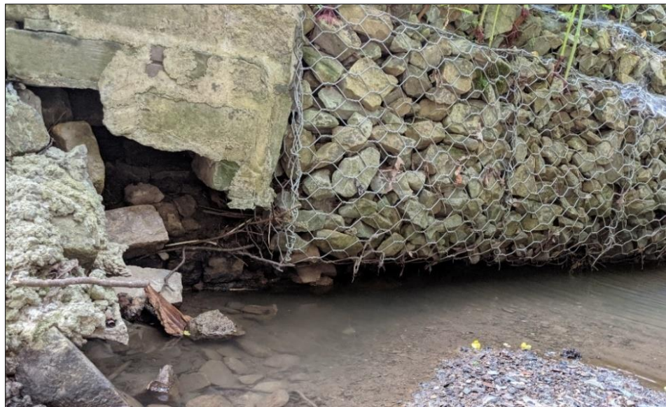
Figure 10-45 - Gabion Wall
