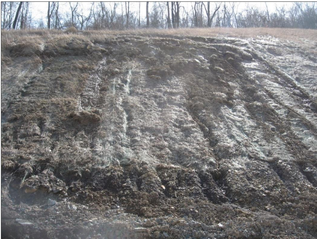
Figure 10-97 - Seepage and erosion gullies formed on the slope below the head scarp
