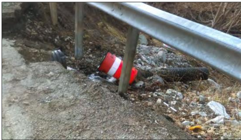
Figure 8-4 - Separated underdrain causing excessive slope erosion leading to a landslide which comprised the shoulder of a roadway (PennDOT District 11)
