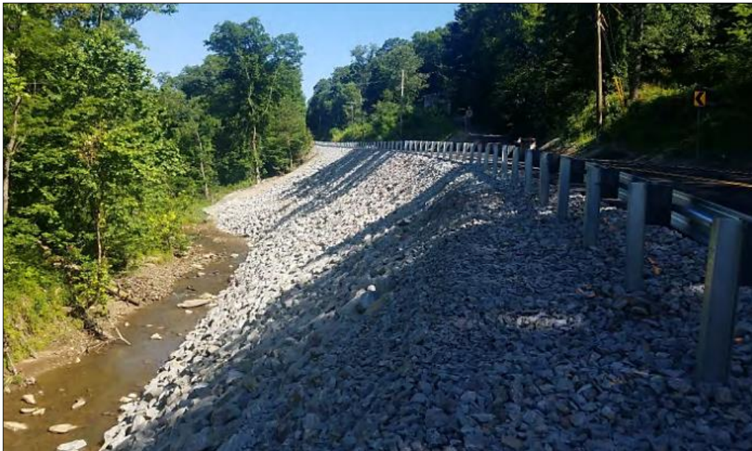
Figure 10-30 - Rock Slope Armoring
