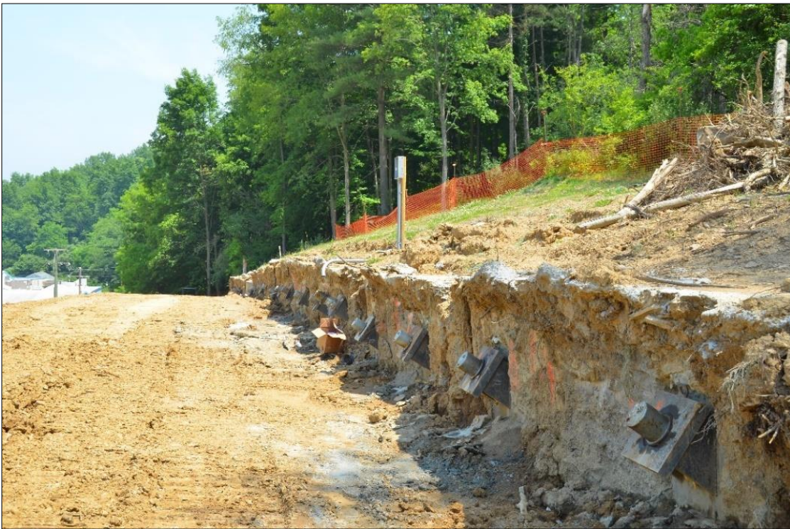
Figure 10-71 - Example Buried Panel Wall with Tiebacks, Anchors Tested, Stressed, Locked Off, and Capped
