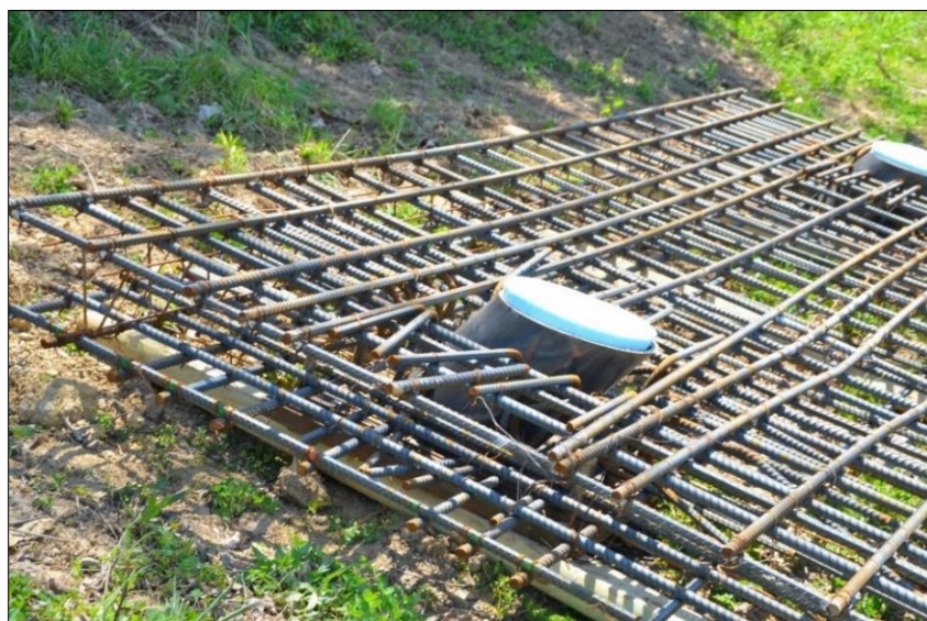
Figure 10-67 - Example Buried Panel Wall with Tiebacks, Rebar Cage with Anchor Sleeve, and Styrofoam Blockout
