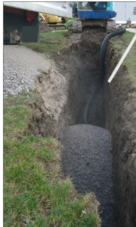
Figure 10-93 - Interceptor (French) Drain
