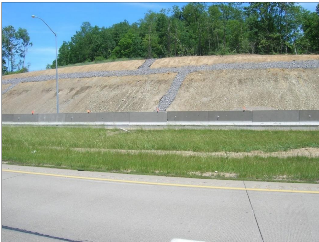
Figure 10-100 - Finger Drains on Slope
