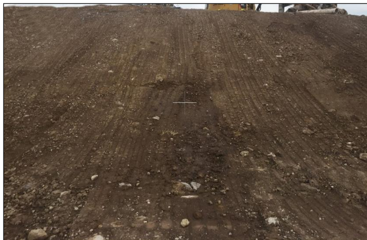
Figure 8-7 - Seepage observed on slope
