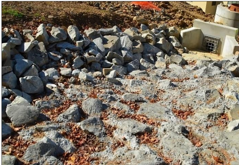
Figure 10-90 - Grouted Rock-Lined Ditch
