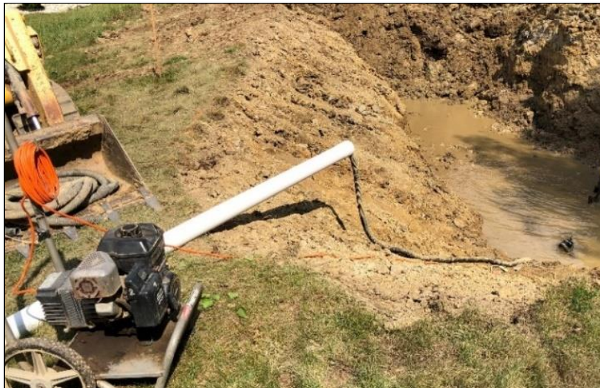
Figure 4-1 – Mitigation effort for a rotational slide caused by excess pore water pressure at the toe of slope; toe key elevation, as shown, intercepted the water bearing Uniontown limestone member
