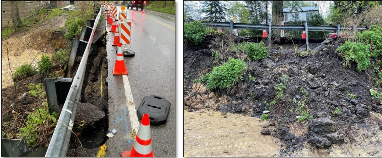
Figure 10-10 - Rock-Fill Buttress Example - Active Slope Failure Looking Down Roadway (left) and Upslope from Toe (right)
