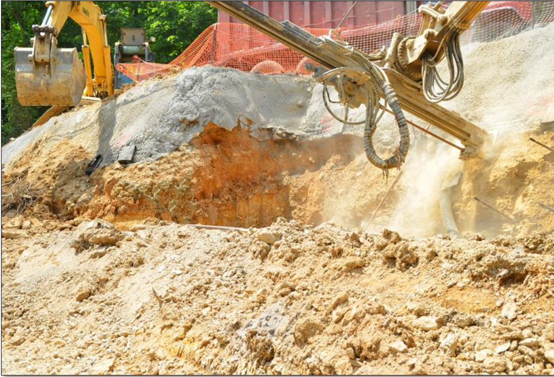
Figure 10-75 - Soil Nail Drilling
