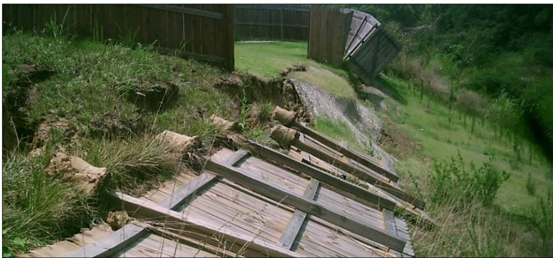
Figure 10-24 - Erosion Gullies in Loamy Soil
