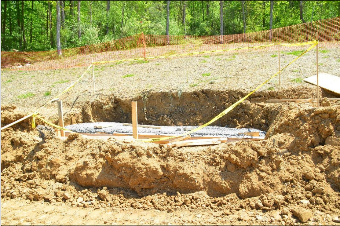
Figure 10-68 - Example Buried Panel Wall with Tiebacks, Trench After Rebar Cage is Set and Concrete is Placed Neat
