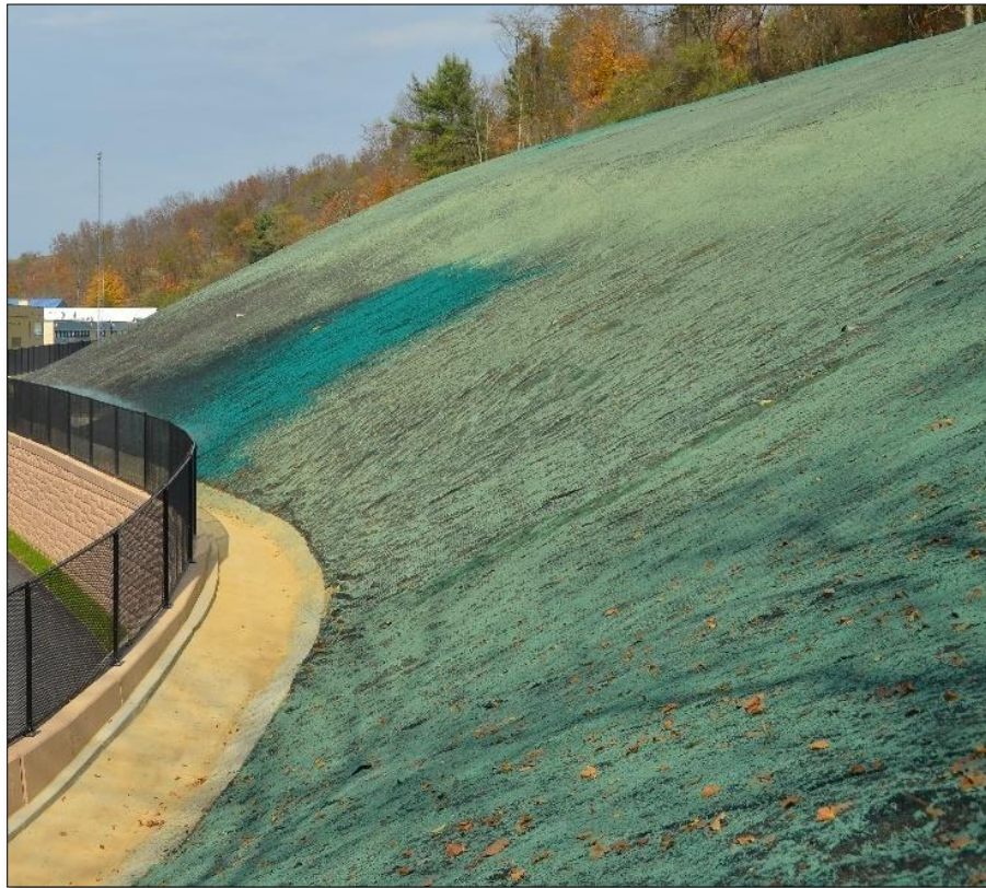
Figure 10-28 - Turf Reinforcement and Hydroseed to Installed Repair and Stabilize Slope
