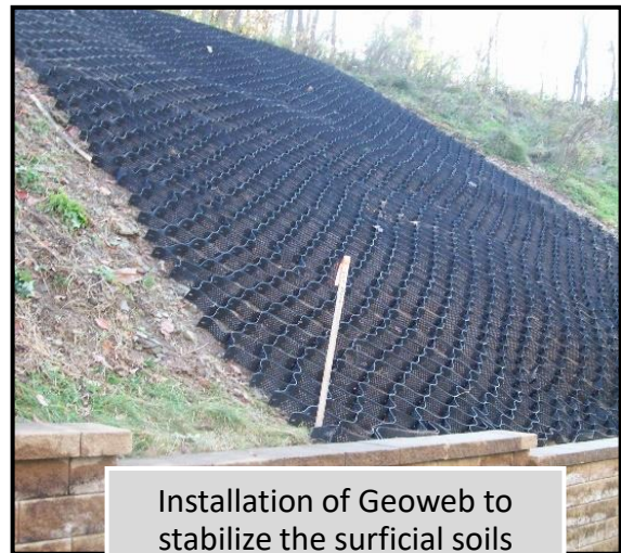
Figure 8-11 - Geoweb installation
