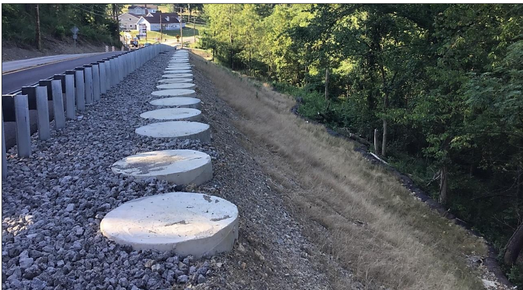
Figure 10-60 - Tangent Piles (PennDOT District 11)
