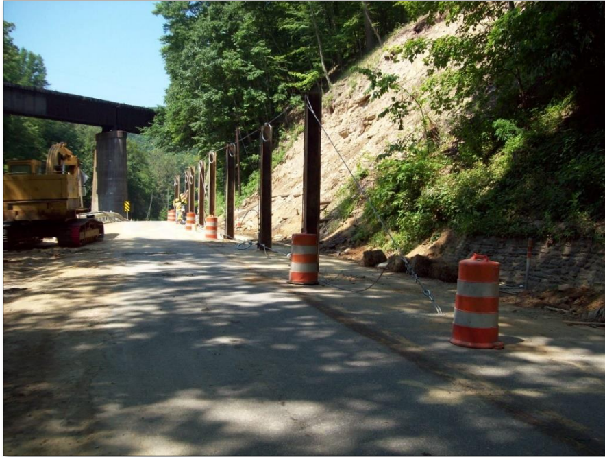
Figure 10-115 - Debris Flow Fence Installation
