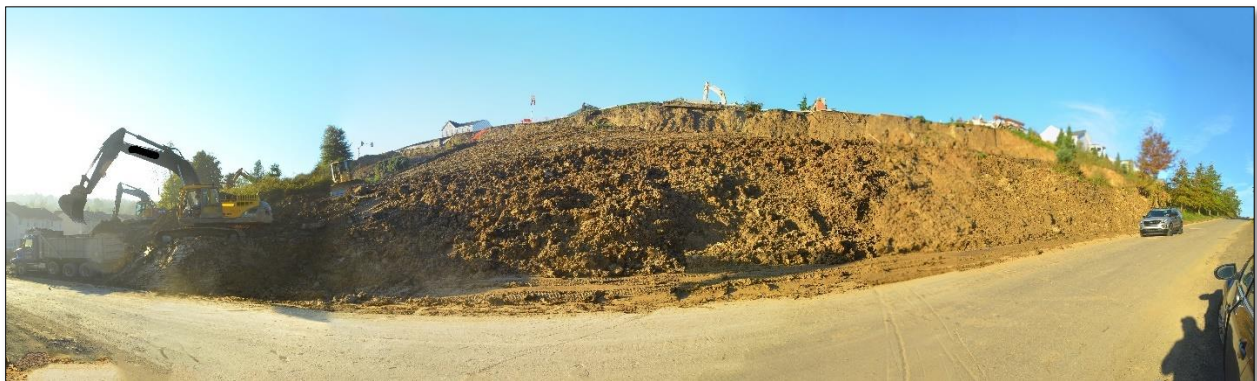
Figure 10-3 - Removal Example Massive Landslide
