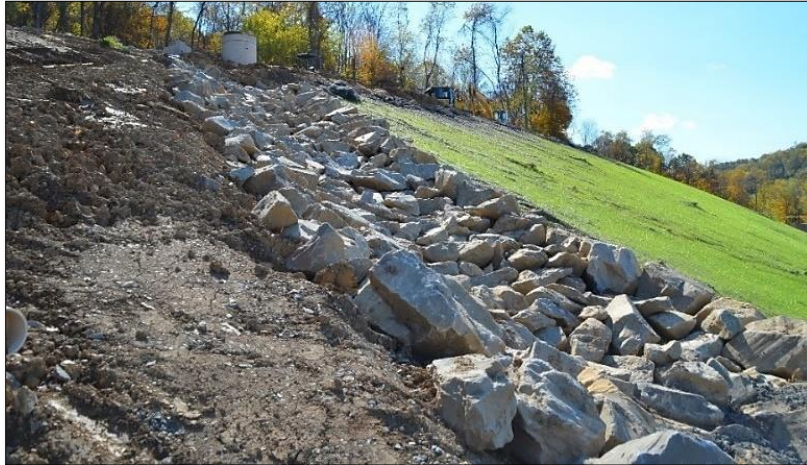
Figure 10-89 - Rock Lined Ditch
