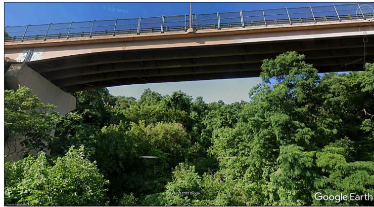
Figure 10-4 - “Bridging” Example Aerial View of McArdle Roadway Spanning over Landslide, Pittsburgh, PA [60]
