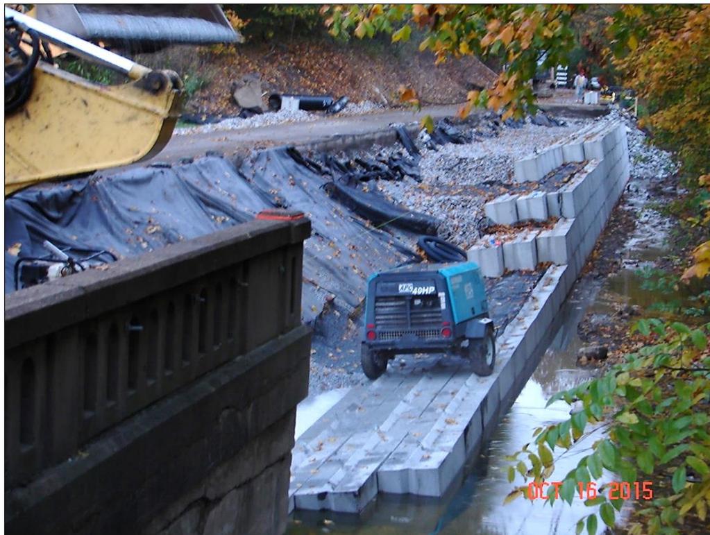
Figure 10-46 - Modular Block Wall Installed for Landslide Repair in Washington County, PA (PennDOT District 11)
