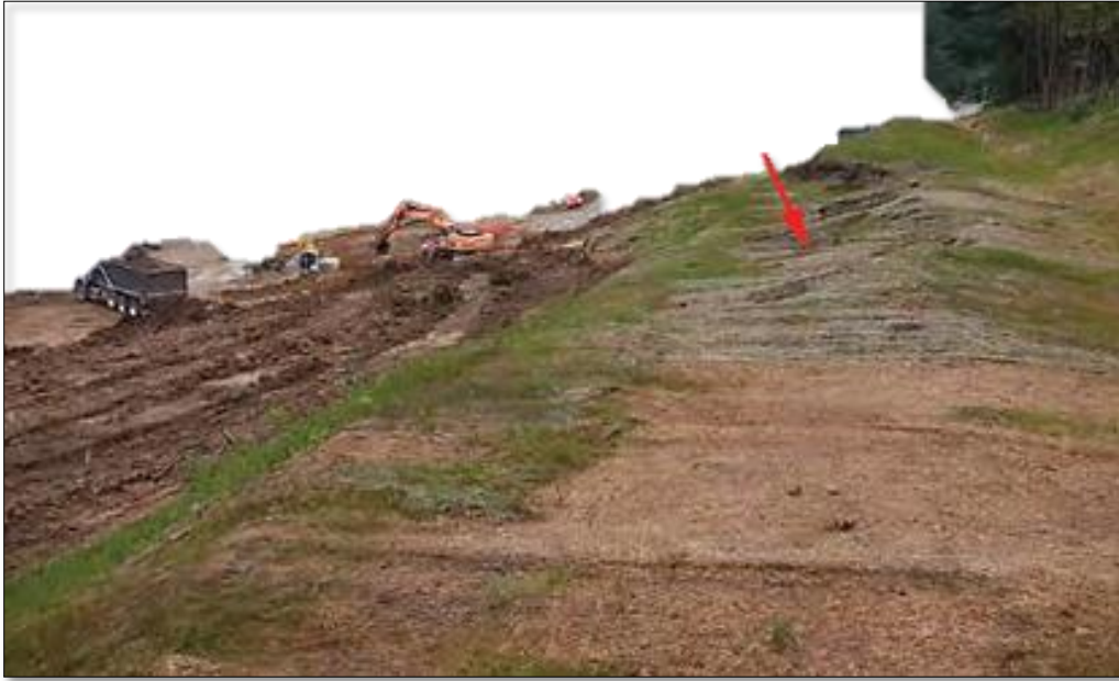
Figure 10-27 - Head Scarp of Carpet Slide
