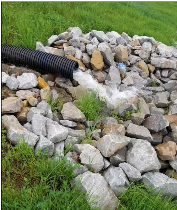
Figure 8-8 - Rip Rap protection at drain outlet (left)
