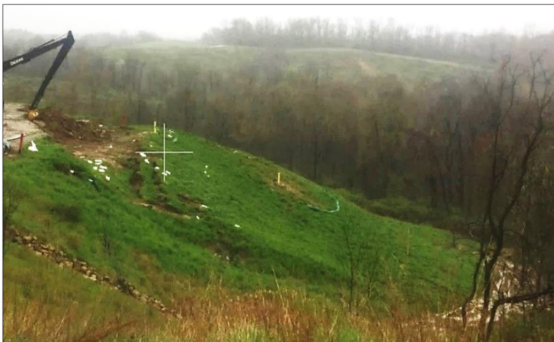
Figure 10-107 - Partial Unloading of Slide Mass
