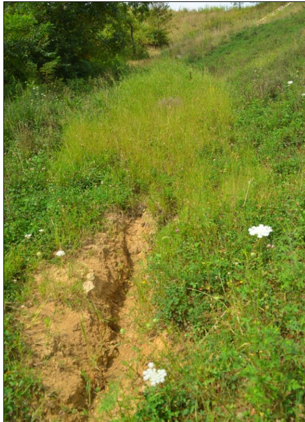
Photograph 2. Embankment Toe, Erosion Rill Looking West
