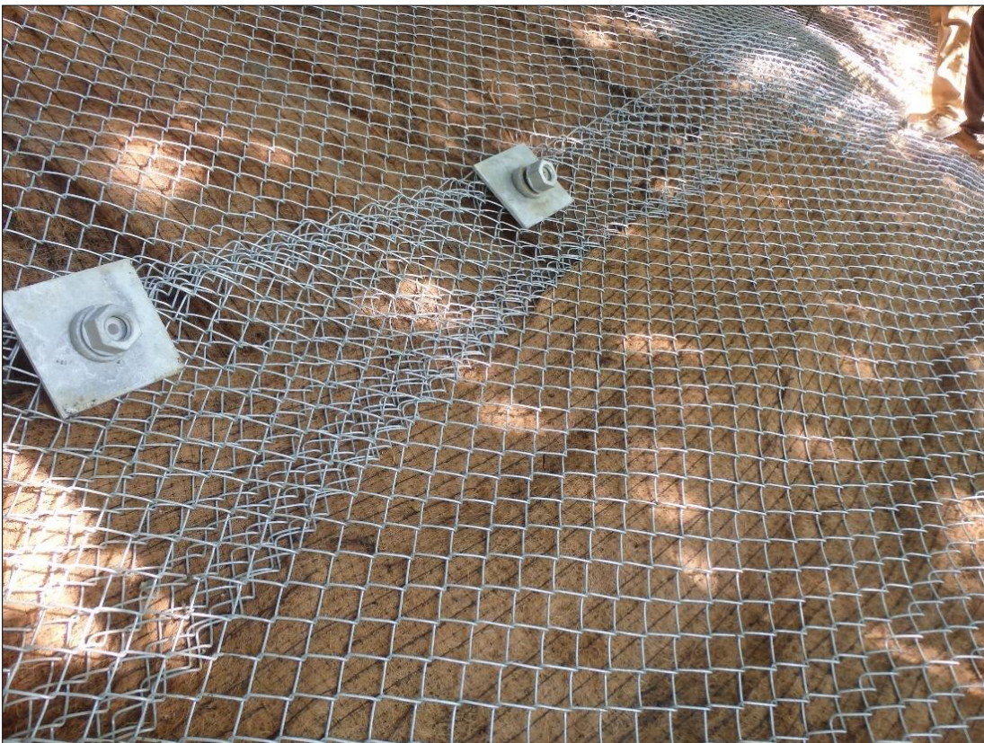
Figure 10-76 - Soil Nails and Wire Mesh
