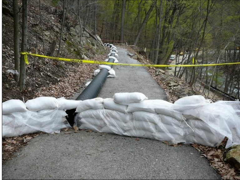
Figure 10-87 - Example of How Sandbags and HDPE Pipe Are Used to Divert Flow from an Active Landslide
