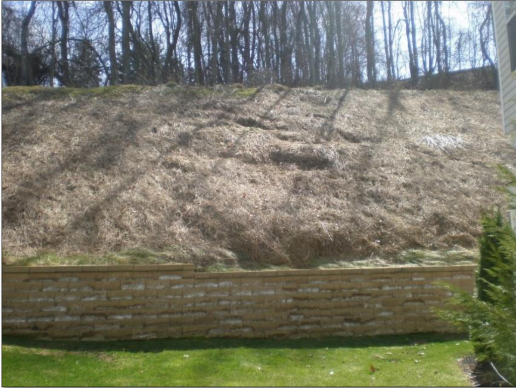
Figure 10-21 - Shallow slope failure
