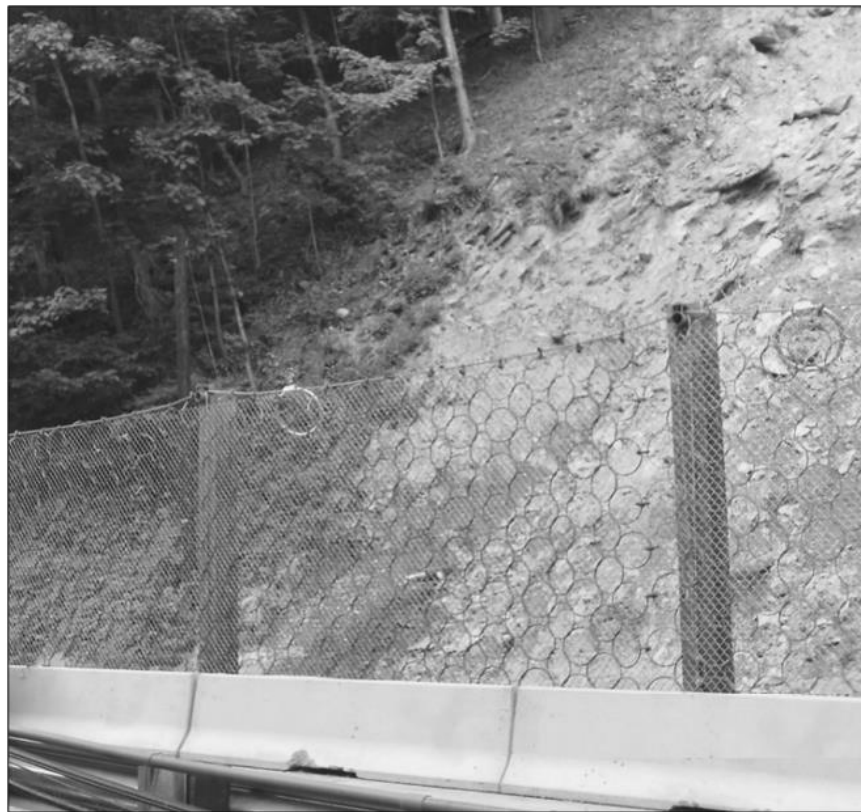
Figure 10-116 - Debris Flow Fence
