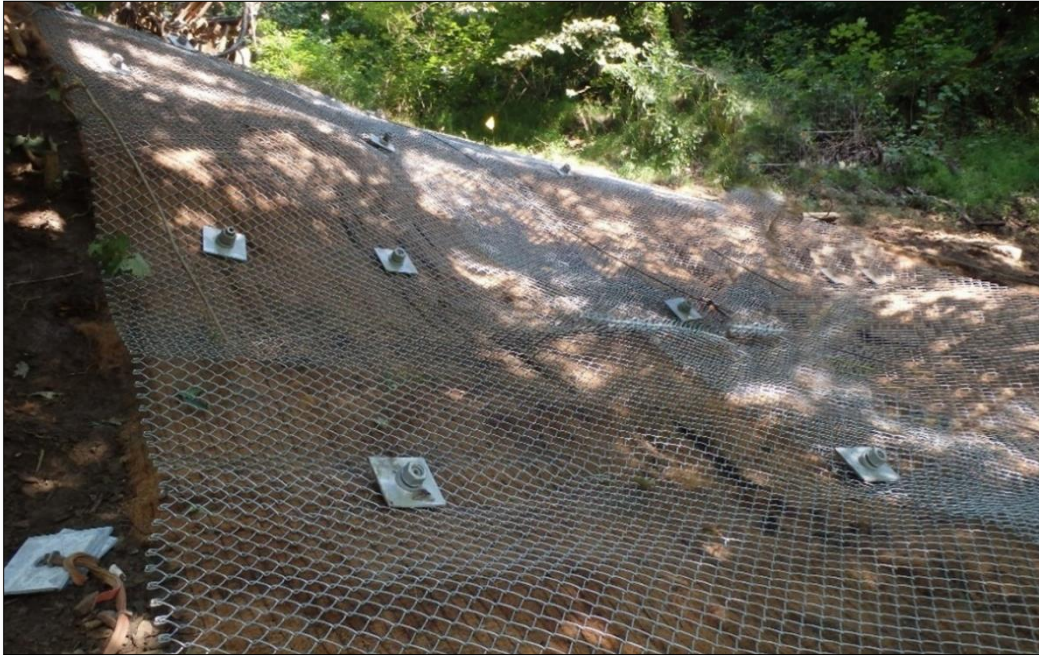
Figure 10-77 - Soil Nails and Wire Mesh
