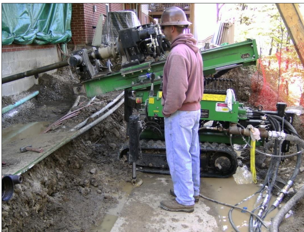
Figure 10-61 - Example Tieback Installation with a Small Duplex Drill on Top of an Existing MSE Wall, Allegheny County
