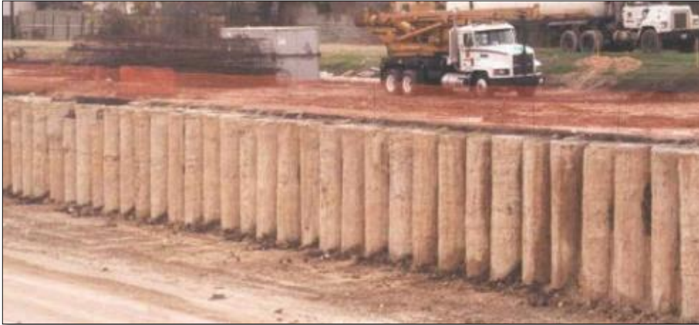
Figure 10-58 - Tangent Pile Wall [48]
