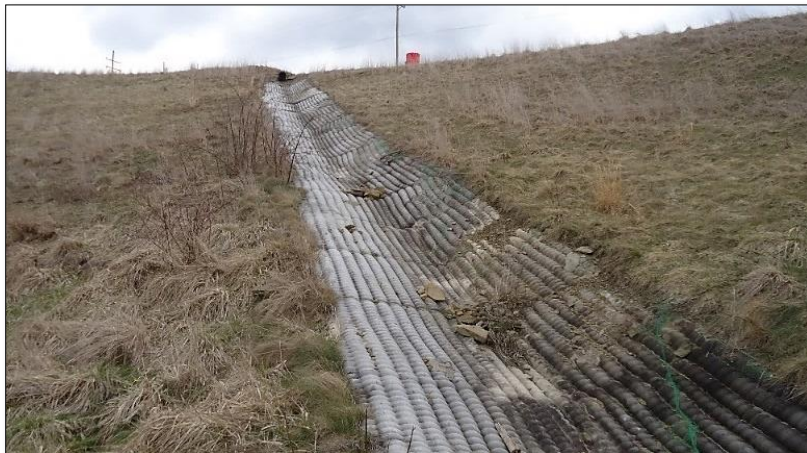
Figure 10-91 - Fabriform Lined Ditch
