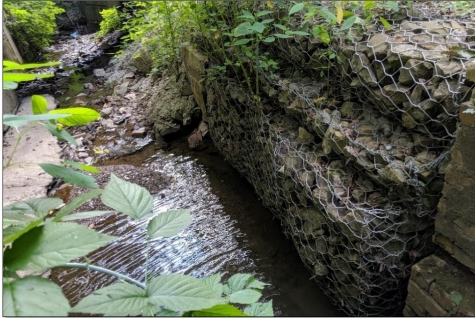
Figure 10-44 - Gabion Wall
