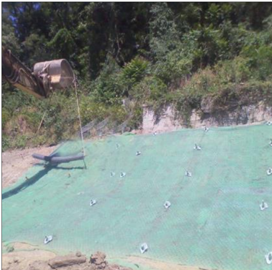
Figure 10-78 - Hydroseeded Soil Nail Slope
