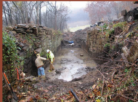
Excavating Lock Chamber
