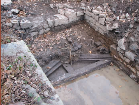
Documentation of Upper and Lower Miter Sills and Gate Remnants
