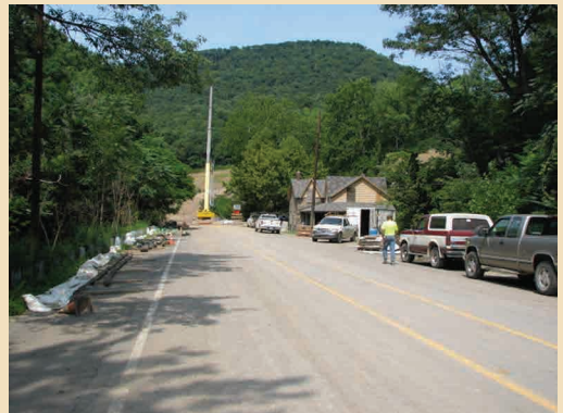
View of Canal Park at beginning of construction, summer 2007
