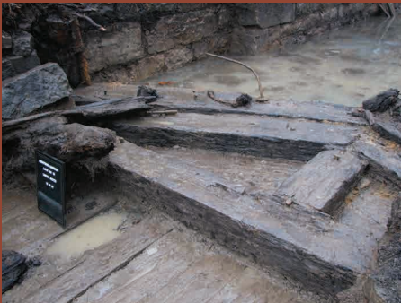
Documentation of Upper and Lower Miter Sills and Gate Remnants
