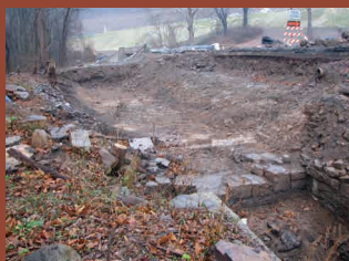
Re-excavation of canal prism at upstream (west) end of lock, January 2008
