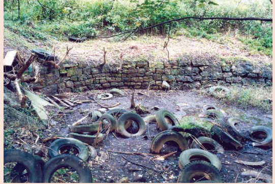
Intact stonework adjacent to the buried Lift Lock No. 14
