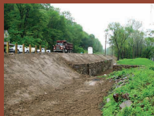
Final grading of prism at upstream end of lock, May 2008
