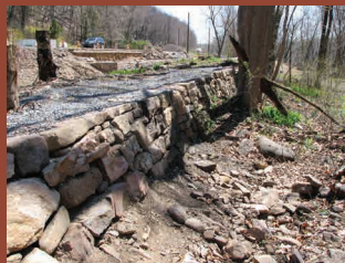
Repaired spillway, May 2008
