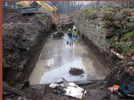
Excavating Lock Chamber
