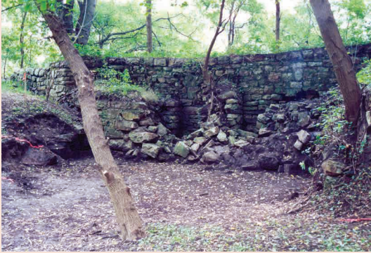
Remains of feeder sluices
