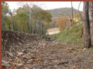
View looking west toward lock after rebuilding of towpath bank, October 2007
