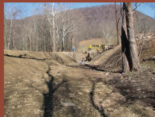
Final grading of towpath, March 2008
