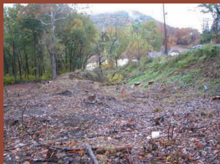
View looking west toward lock after preliminary clearing, October 2007
