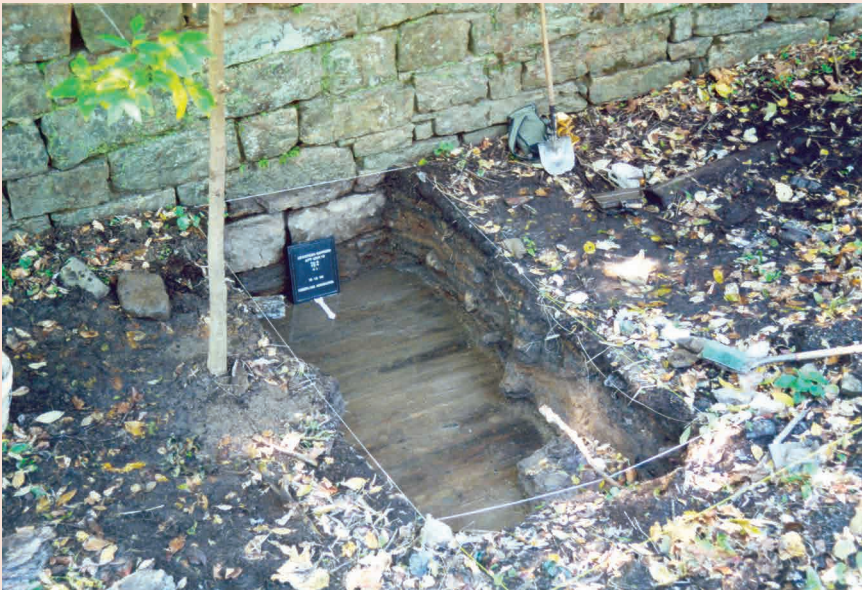
Archaeology exposed the original wood plank floor of the lock
