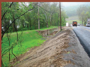
Final grading of berm bank, May 2008
