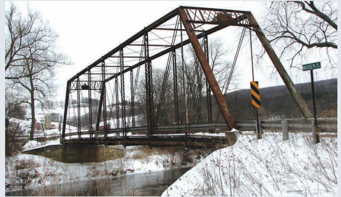
21. Maust Bridge (County Bridge No. 21)
