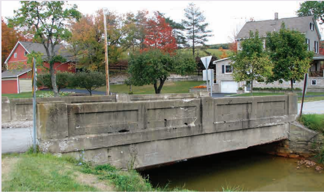
30. Buffalo Creek Bridge
