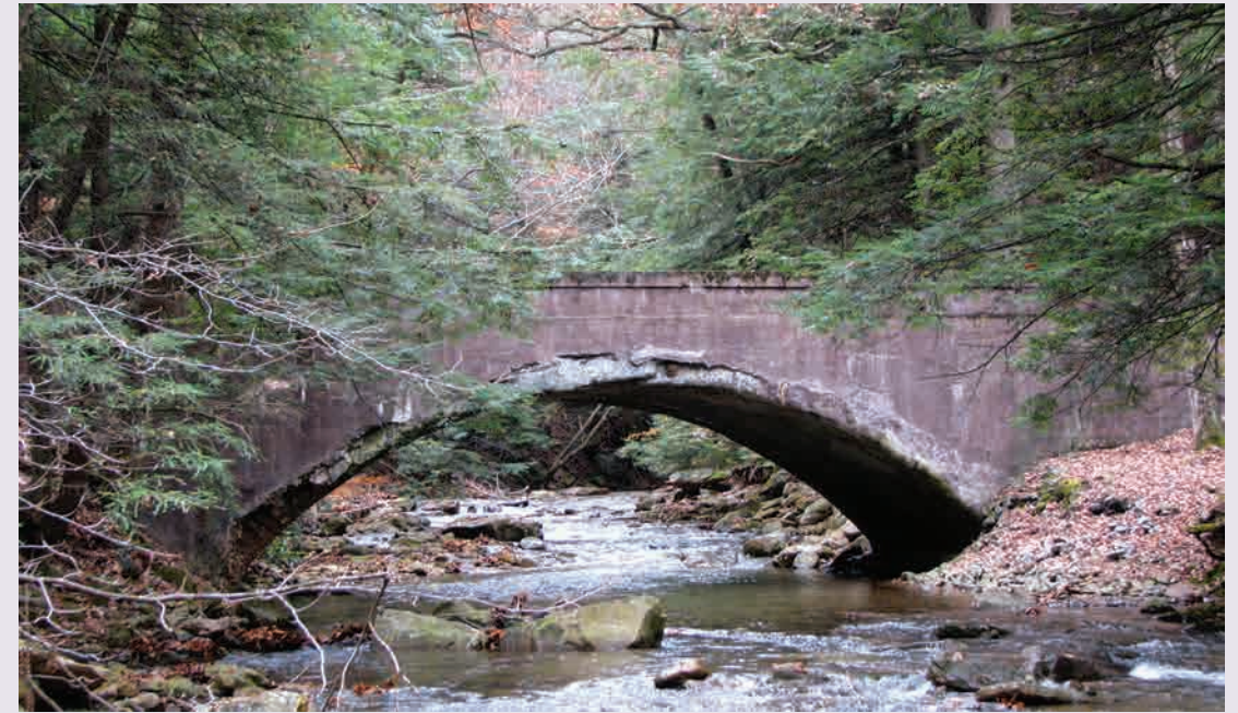
29. Mickey Bridge (County Bridge No. 41)
