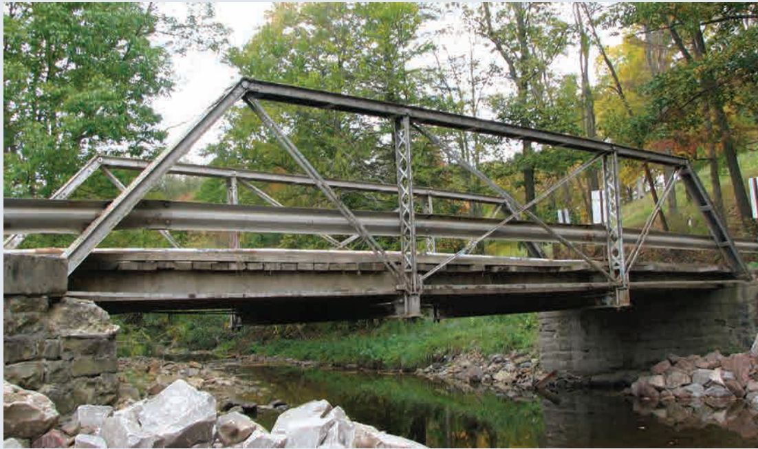
16. Bender Bridge Road Bridge
