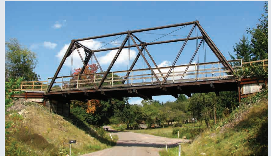
15. W. Bollman and Company Bridge
