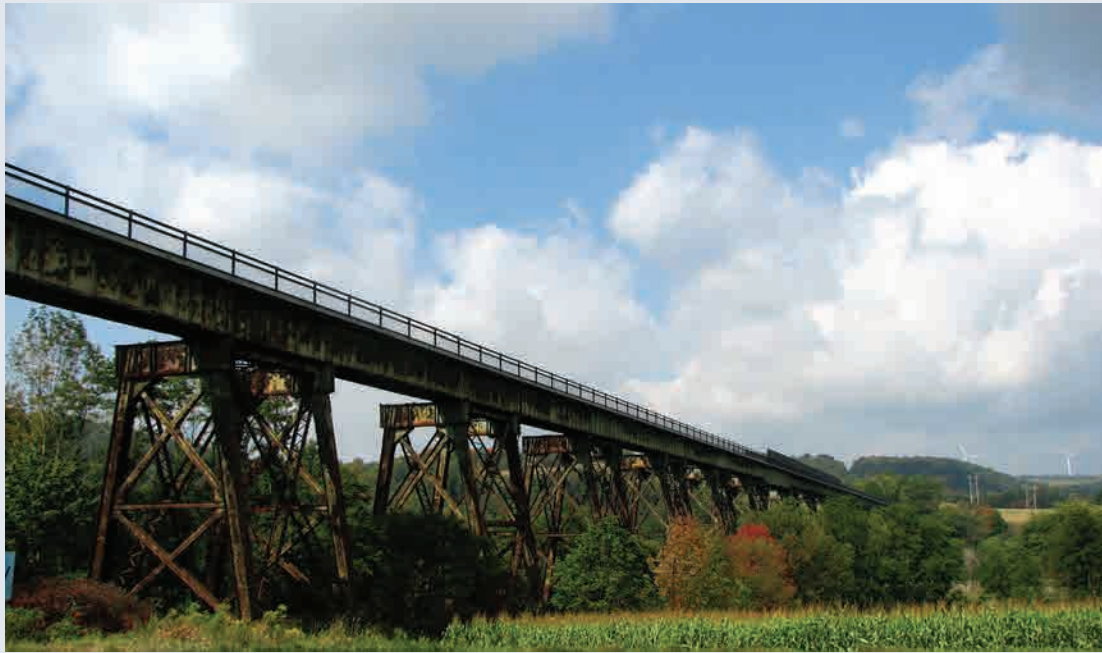
24. Salisbury Junction Viaduct
