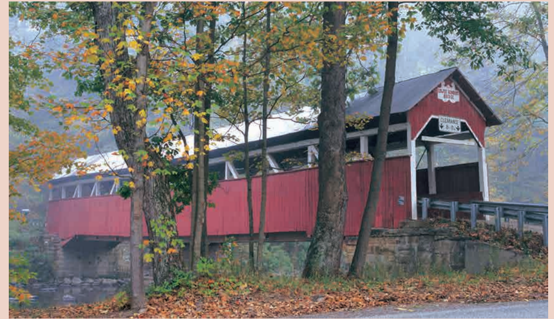
13. Lower Humbert / Faidley Bridge
