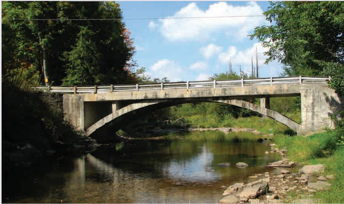
28. Engle Bridge (County Bridge No. 24)
