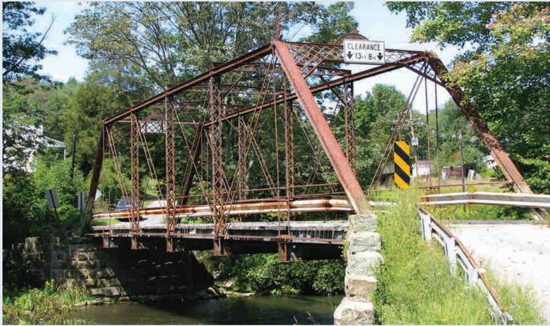
18. Fleegle Bridge (County Bridge No. 48)
