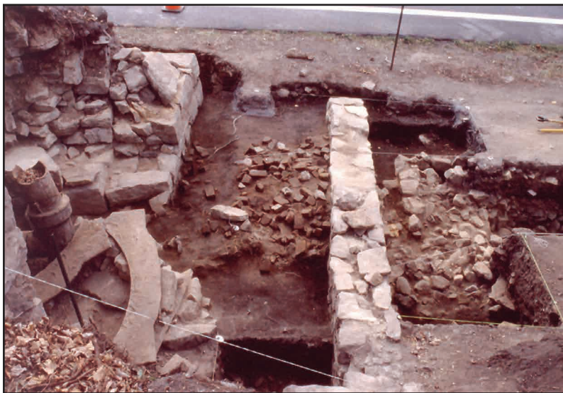
West room at Rockhill Furnace after excavation. Brick rubble (center) and curved iron plates (left) were thrown from top of stack when furnace was dismantled about 1876. Stone rubble (right) was deposited when site was filled and leveled before furnace was built.
