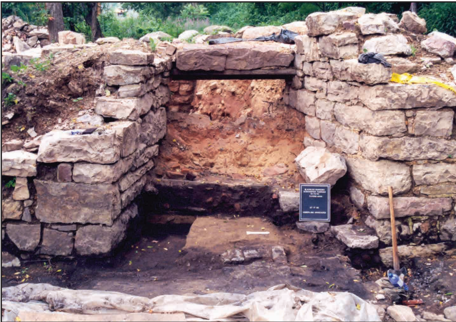
Remains of tuyere arch at Winchester Furnace
