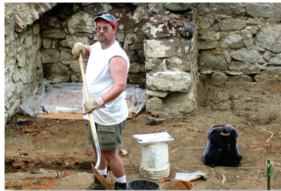
Intensive excavation being conducted at Site 7NC-B-11, a historic farm complex in Wilmington, Delaware.
