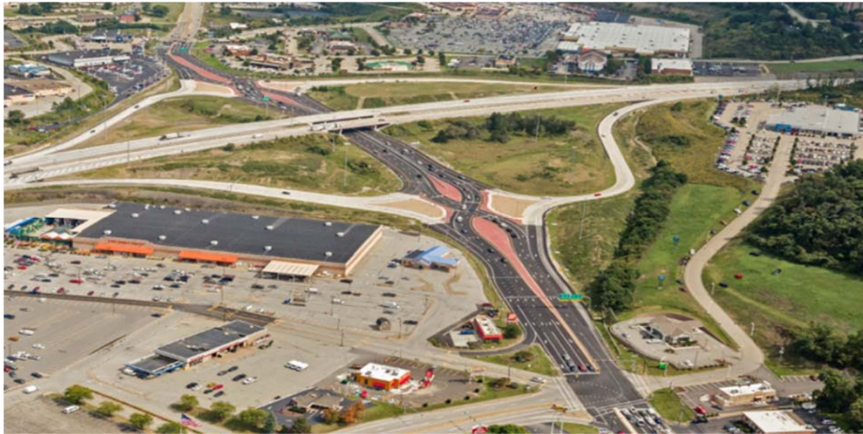
FIGURE 16: US 19/I-70 DIVERGING DIAMOND INTERCHANGE, SOUTH STRABANE TOWNSHIP
