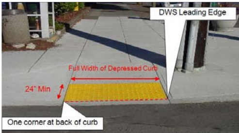
DETECTABLE WARNING SURFACE (DWS) EMBEDDING DETAIL
