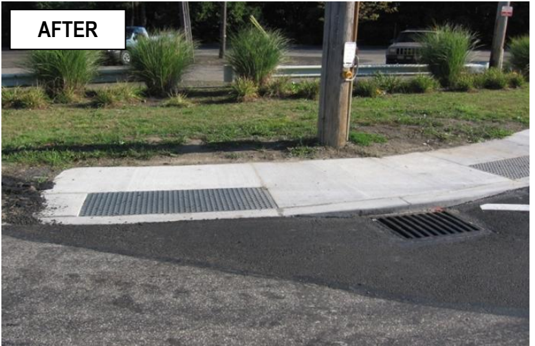
Adjacent Type 2 curb ramps.
