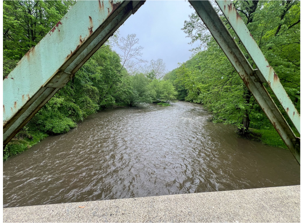
Standing on the Bridge Looking Upstream
