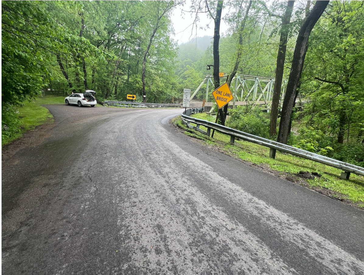
Near Approach of Old Mercer Road Looking East
