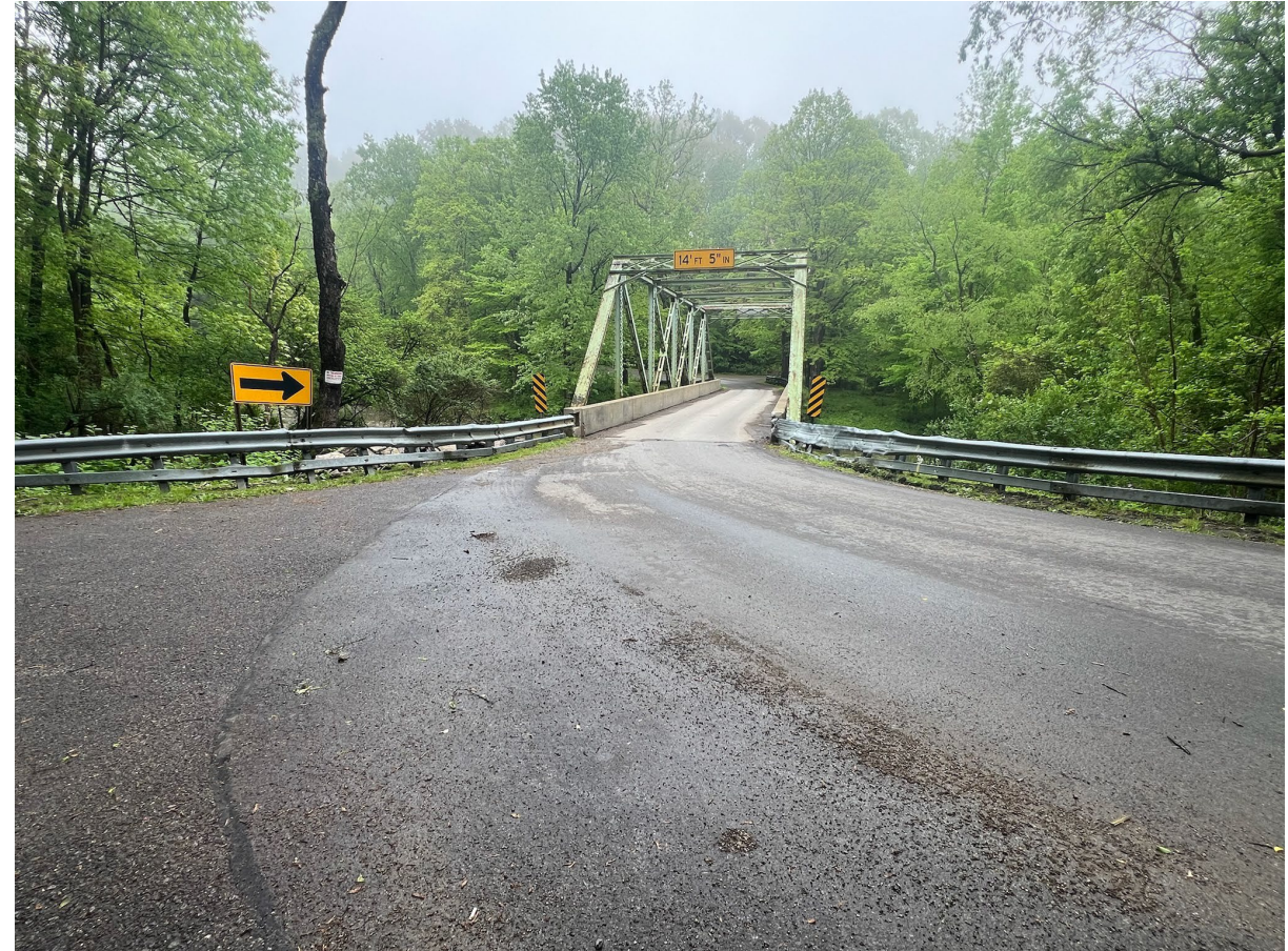
Far Approach of Old Mercer Road Looking North
