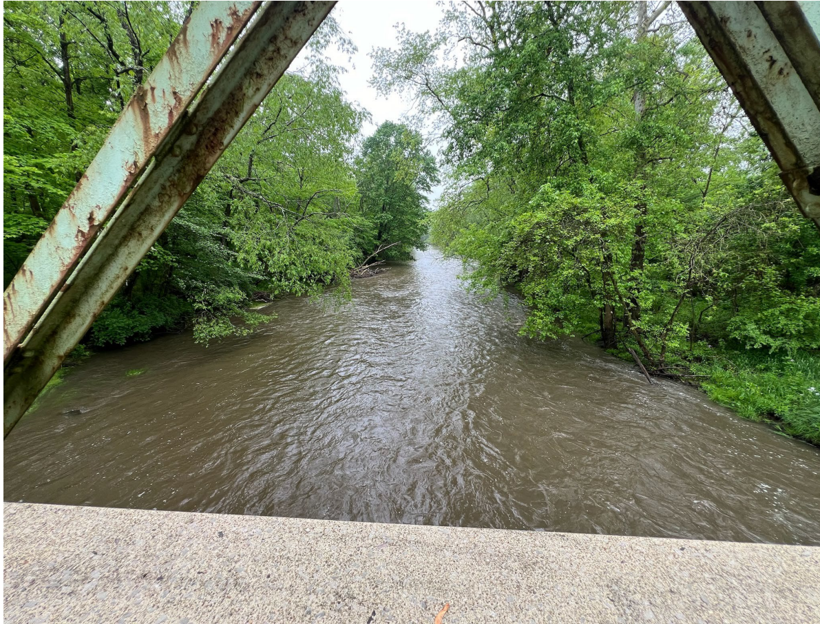
Standing on the Bridge Looking Downstream
