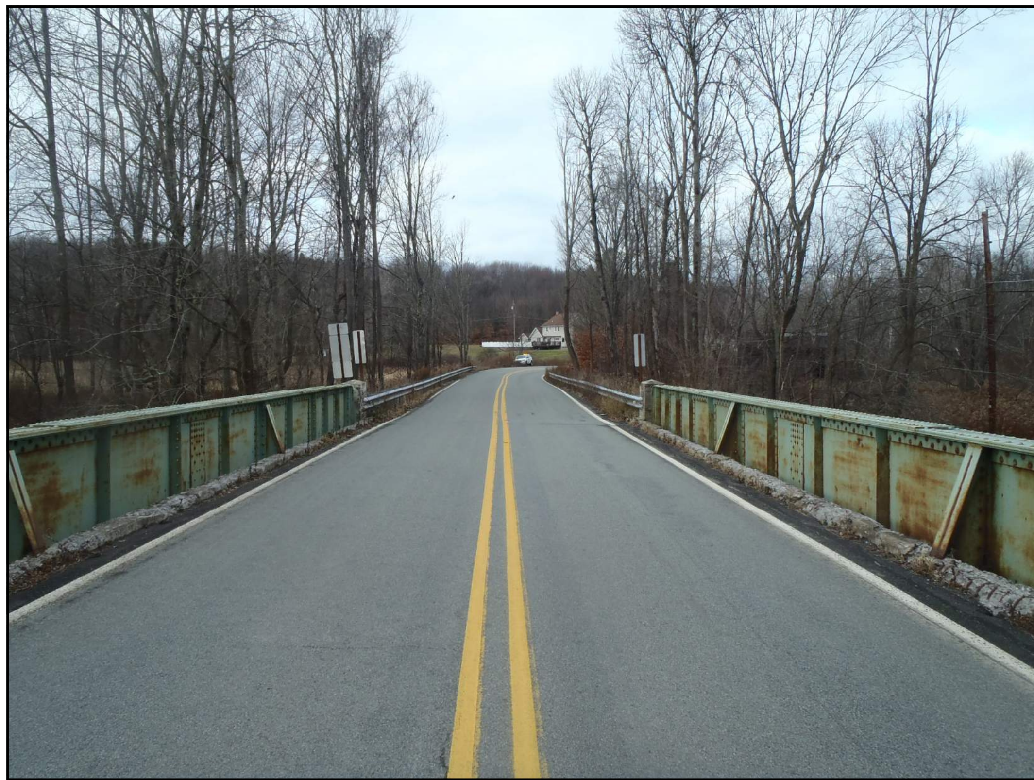
View atop the existing bridge looking North toward the northern approach
