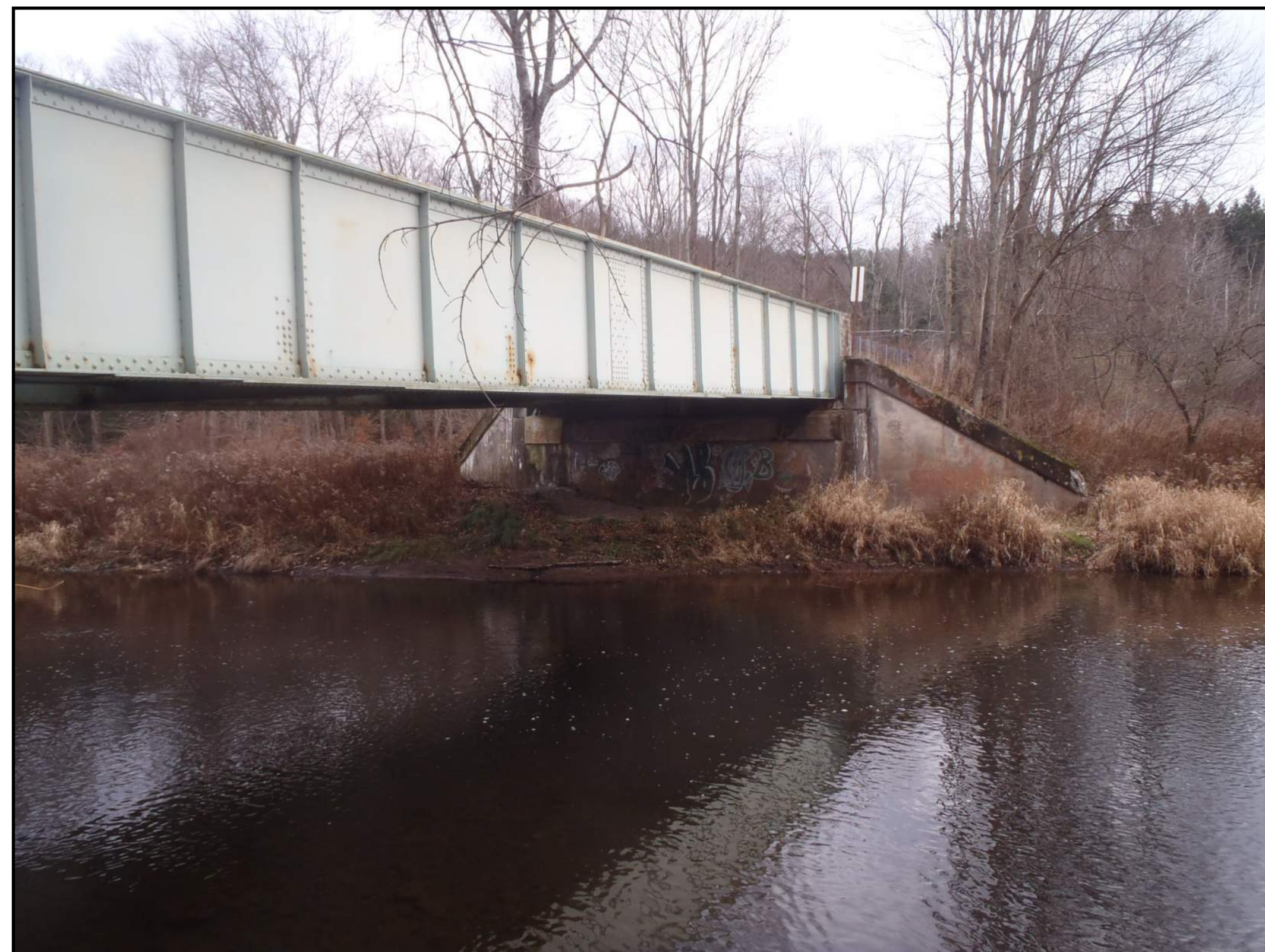
Upstream elevation of the existing bridge (looking Southeast)
