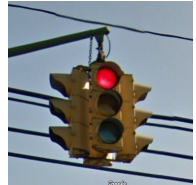
EXISTING TRAFFIC SIGNAL HEAD AT FIFTH STREET
