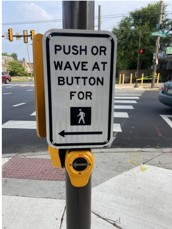
Accessible Pedestrian Signal (APS) Push Button
