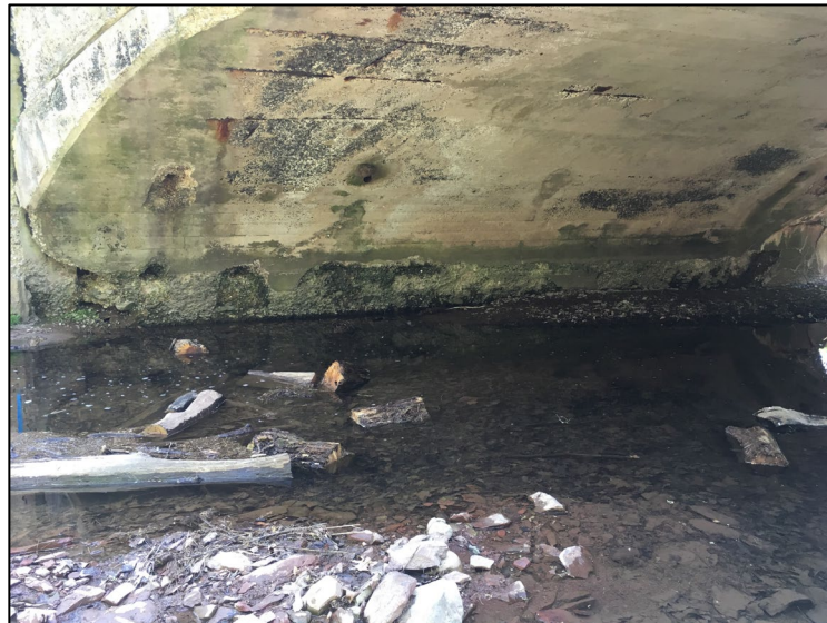
Underside of arch looking northeast
