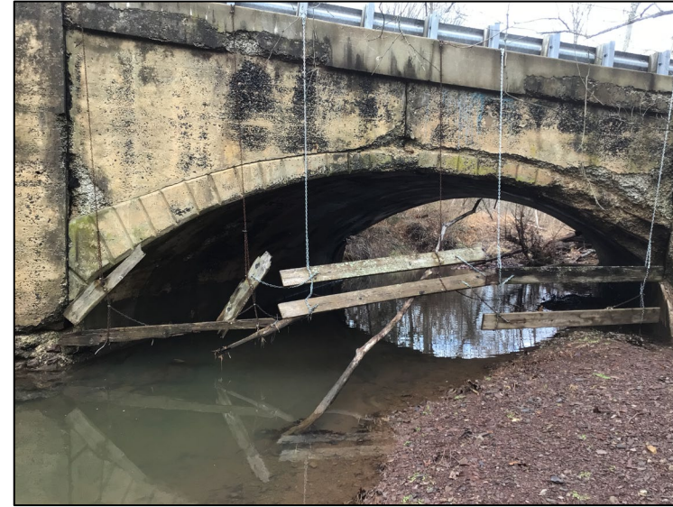
Overview of concrete arch on downstream side of bridge
