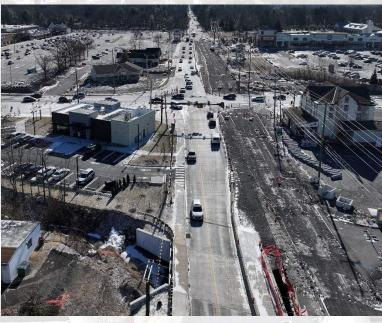
Demolition of the old culvert at 2<sup>nd</sup> Avenue has been completed, and excavation of the old concrete roadway and installation of the new storm drainage are currently ongoing, on the west leg of Skippack Pike.
