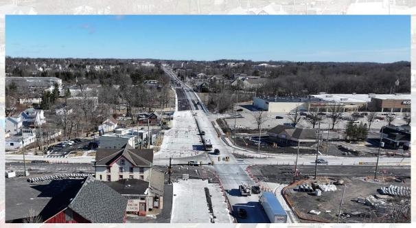
**On U.S. 202,** construction of the new concrete pavement within the Skippack Pike intersection will be a phased operation, requiring traffic on U.S. 202 to be shifted from the northbound side of the road to the southbound side of the road, in order to complete the work.
