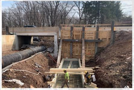
On U.S 202 between Germantown Pike and Jefferson Crossing Boulevard, the contractor completed the construction of the temporary sediment basin and has started construction of the new drainage systems on the southbound side of the roadway.
