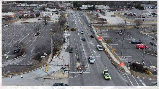
On U.S. 202 between Germantown Pike and Township Line Road, the contractor has completed the construction of the footing slabs for the new noise barrier wall between U.S 202 and Dekalb Boulevard. This spring, the contractor will continue with the construction of the cast-in-place stem walls, followed by the installation of noise wall posts and panels.
