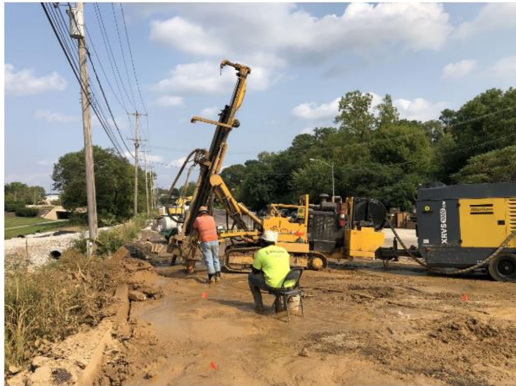
Battered grout hole drilling near overhead utilities
