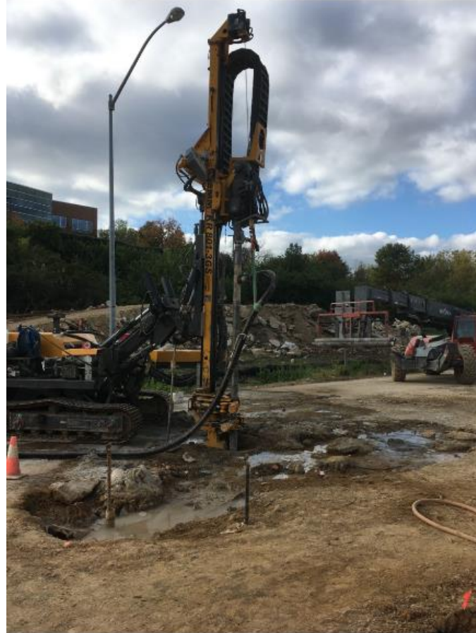
Vertical grout hole drilling
