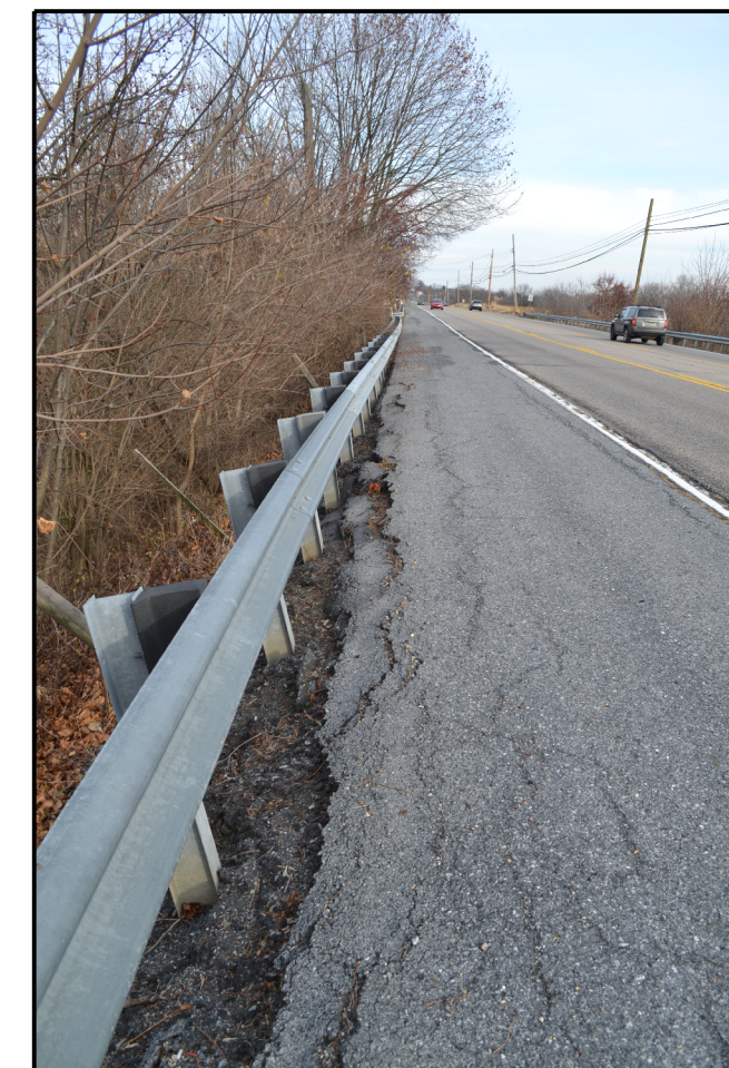
SHOULDER RECONSTRUCTION AREA (LOOKING WEST)
