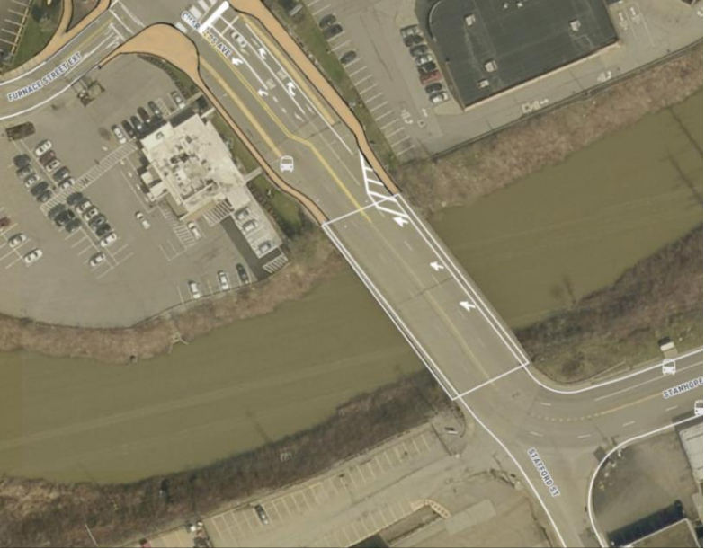
Tie-in to Existing Lanes on Bridge
