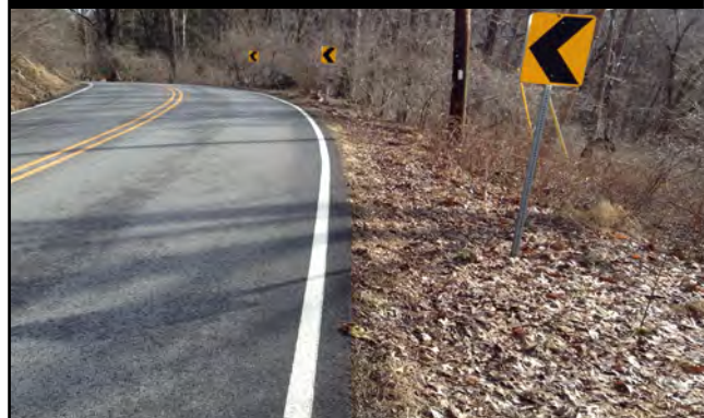
Figure F-4. Chevron Signs on Outside of Curve
