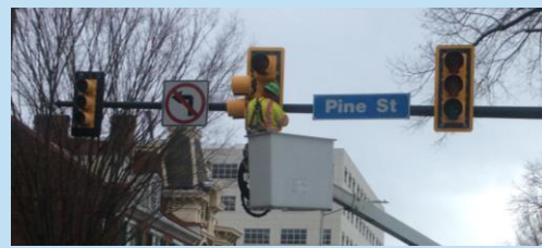
Upgrading 8" to 12" signal heads
