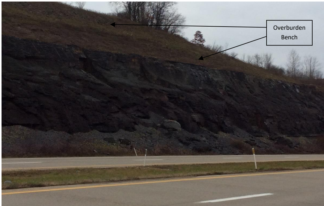
Figure 8.6.1-1 – Example of an Overburden Bench
