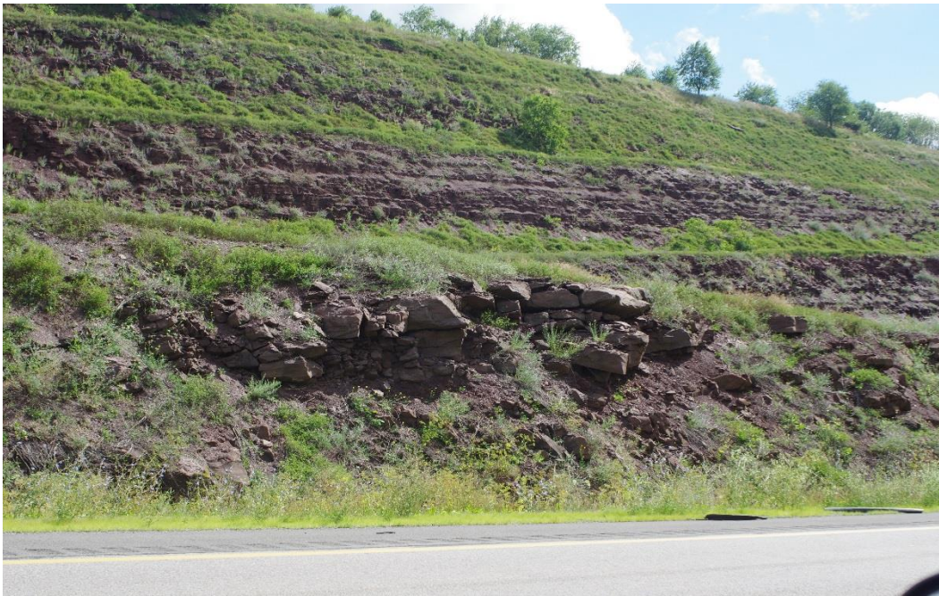
Figure 8.6.2-1 – Example of a Geotechnical Bench
