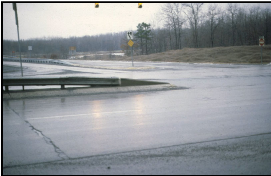
Sloped Concrete on a W-Beam System
