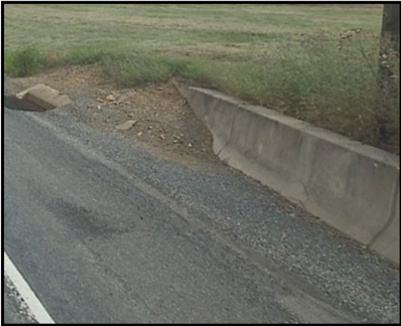
Example of undamaged 1-BIBS for concrete barrier.
