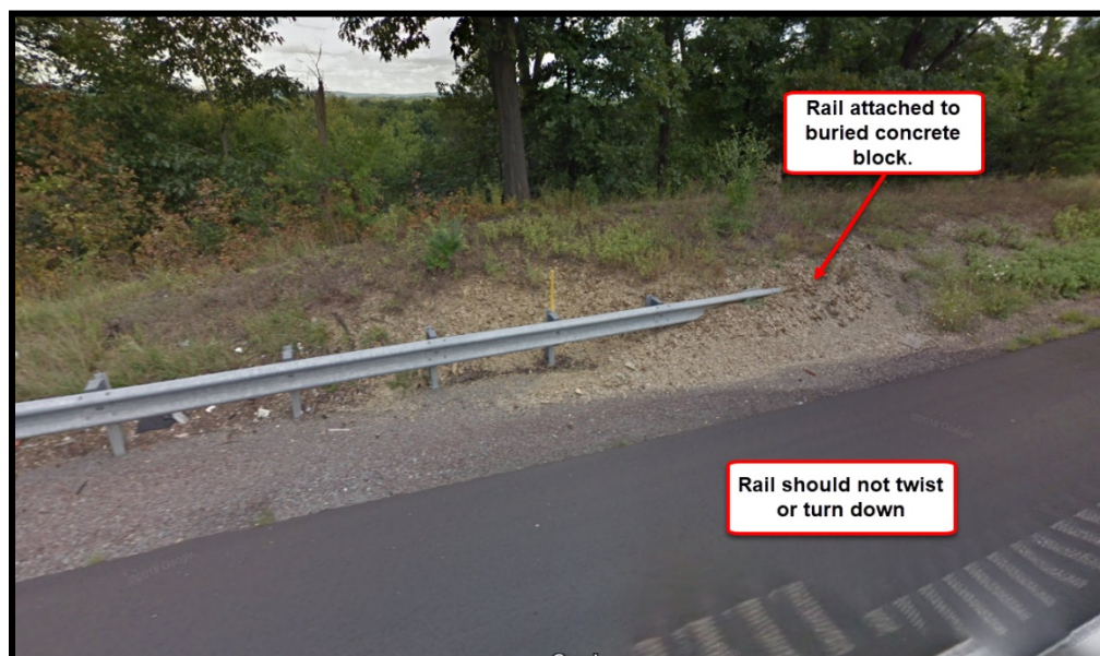
Undamaged Type 1-BIBS for W-Beam Guide Rail
