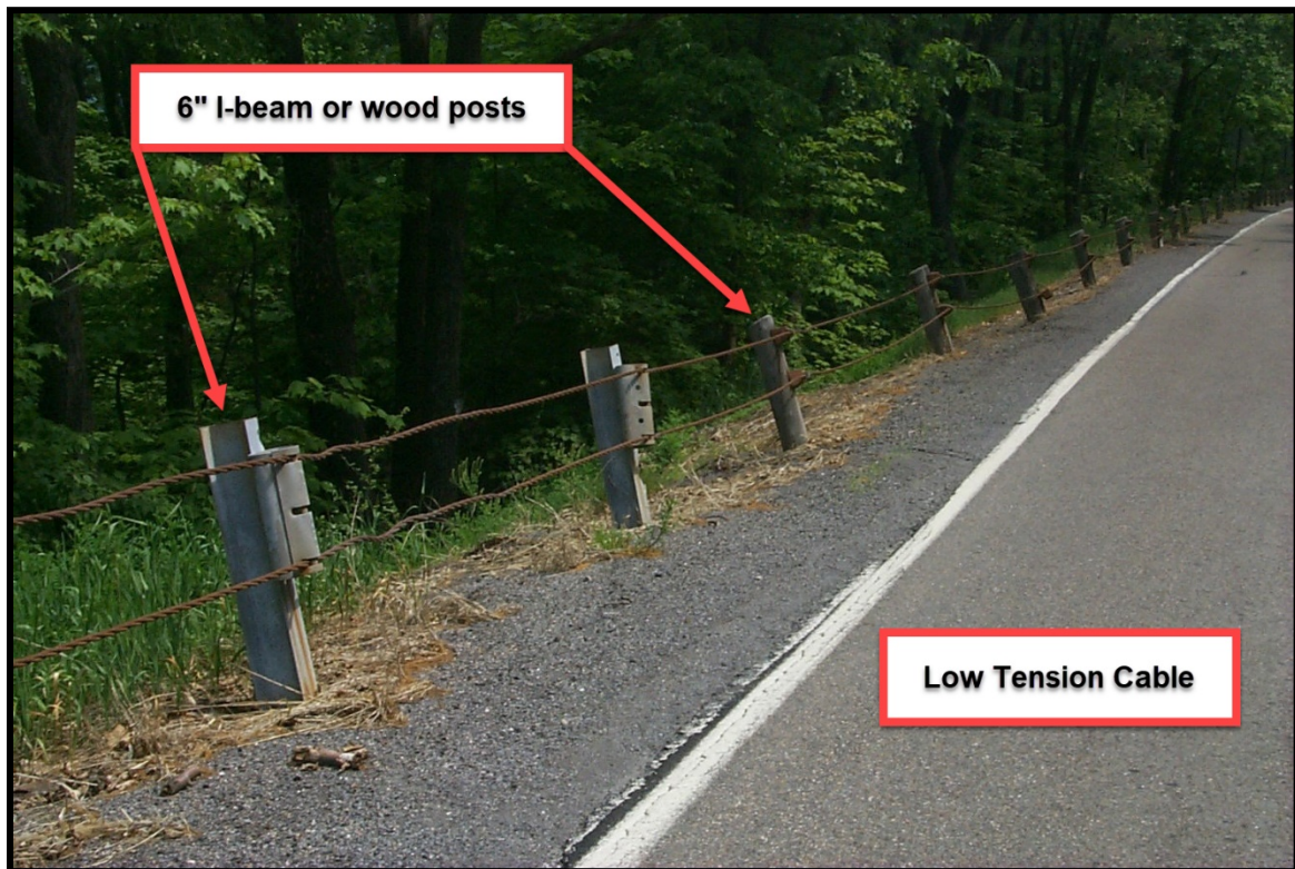
Two Cable Steel Post Strong Post Cable System (6" I-Beams) With Two Cable Wood Post Strong Post Cable System
