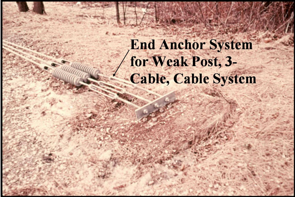
Undamaged Type 1-BIBS for Weak Post, 3-Cable, Cable Guide Rail. Similar for High-Tension Systems
