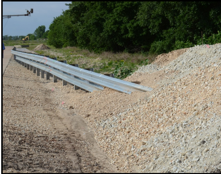
Example of double rail installation buried in back slope (1-BIBS).
