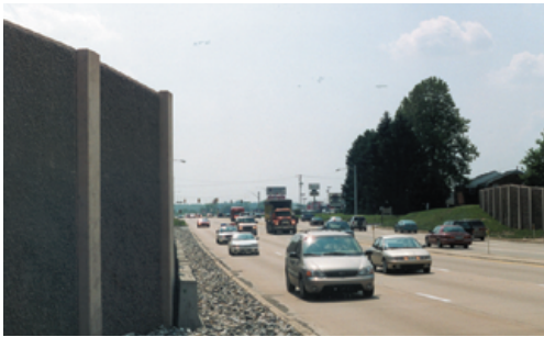
Traffic noise wall along a roadway
