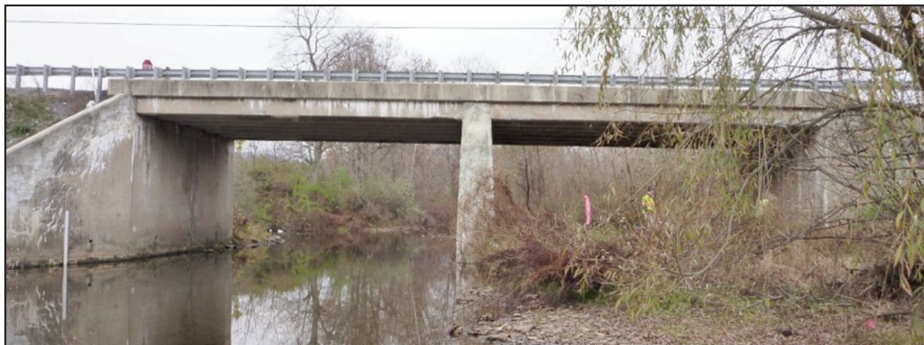
Figure 6: Marsh Creek Bridge
