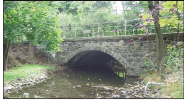
Figure 4: Stone Arch Bridge over Saucon Creek
