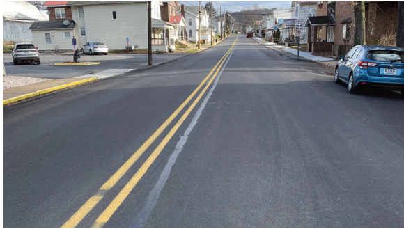
Completed Turnback of SR 1025, now Main Street, in Marion Center Borough, Indiana County
