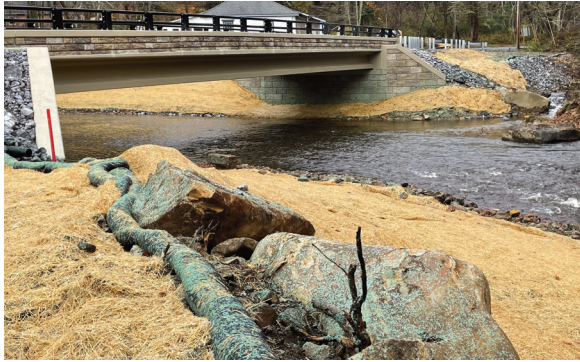
Red Mill Bridge Replacement Project in Blacklick Township, Cambria County.
