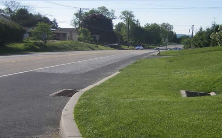
Figure 2.1.1- Conventional installation where enclosed surface storm water facility connects to highway storm water facility.
