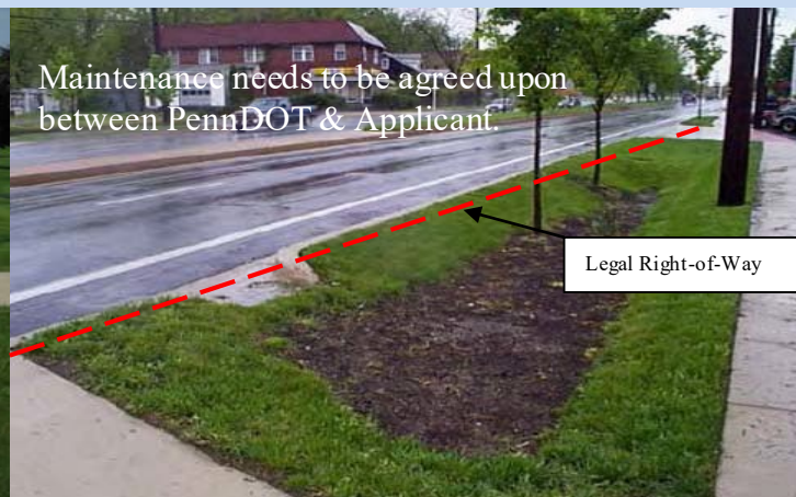
Figure 2.3.2- Alternative installation directs water to an infiltration trench off the right-of-way without the use of inlets and enclosed storm water facilities.
