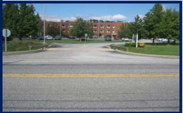
Figure 1.1.2- Culvert conveys water under driveway.
