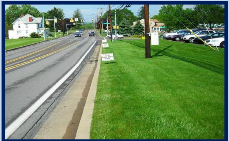
Figure 1.4.2- New enclosed surface storm water installed with curb gutter as part of widening for left turn lane.
