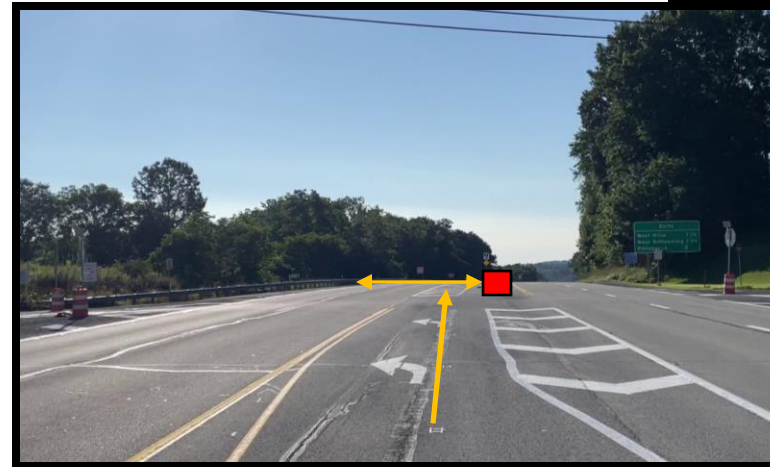
Left turn lanes were shifted to eliminate sight distance conflicts and reduce the amount of time to complete a crossing maneuver
