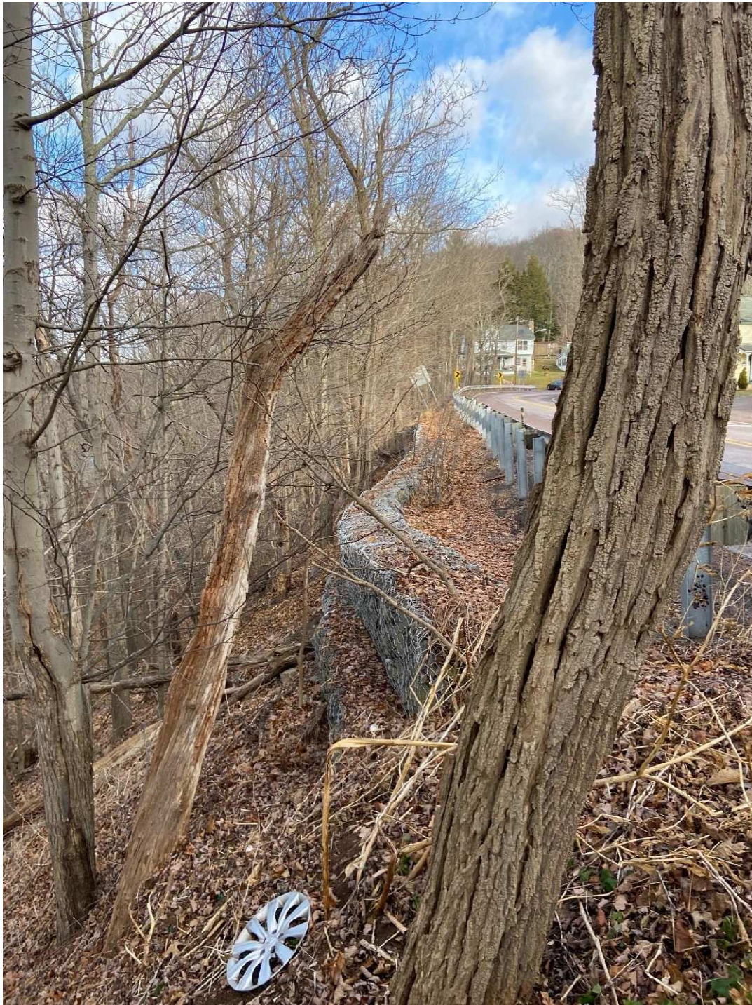
View of SR 940 Existing Gabion Wall, facing north
