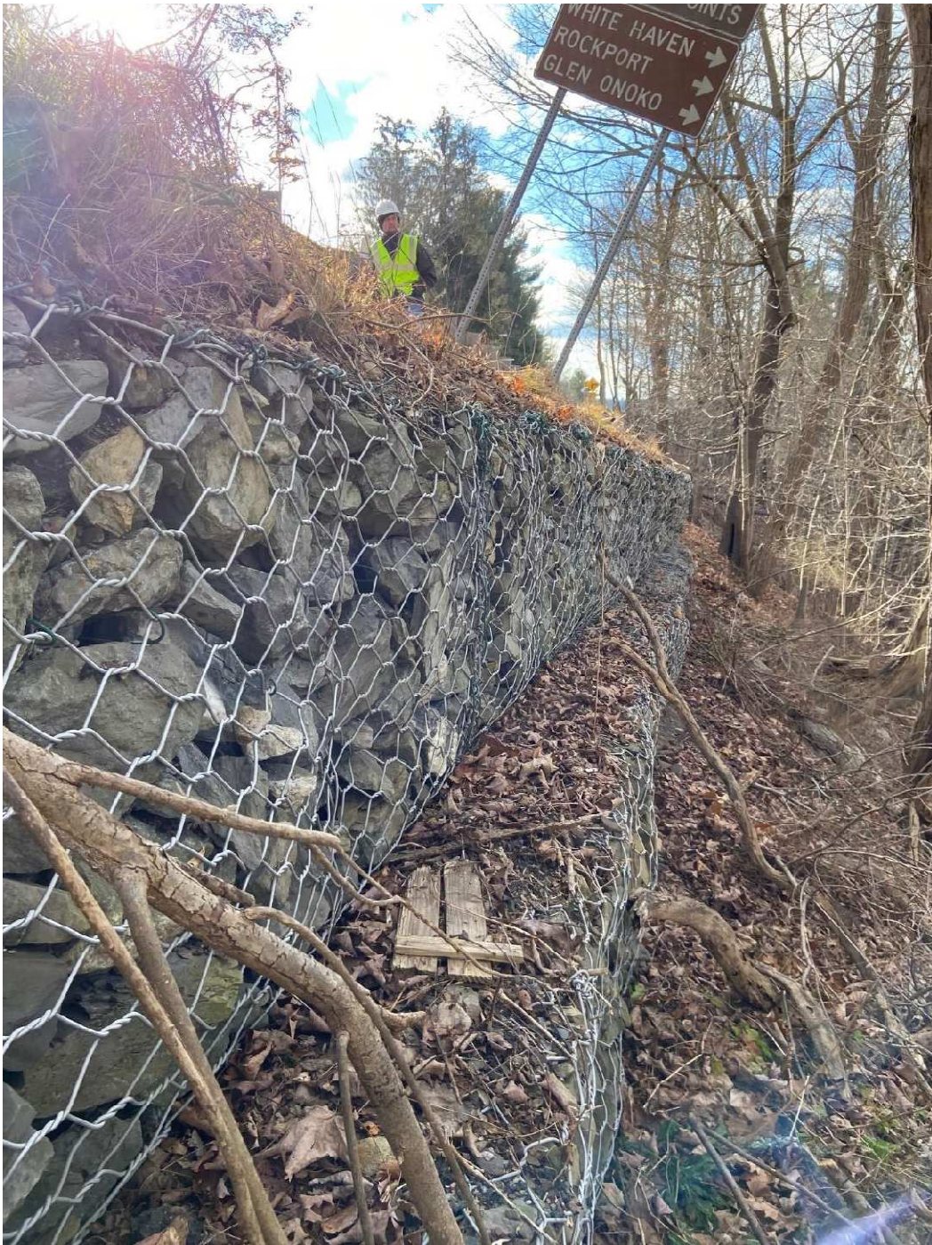
View of SR 940 Existing Gabion Wall, facing south
