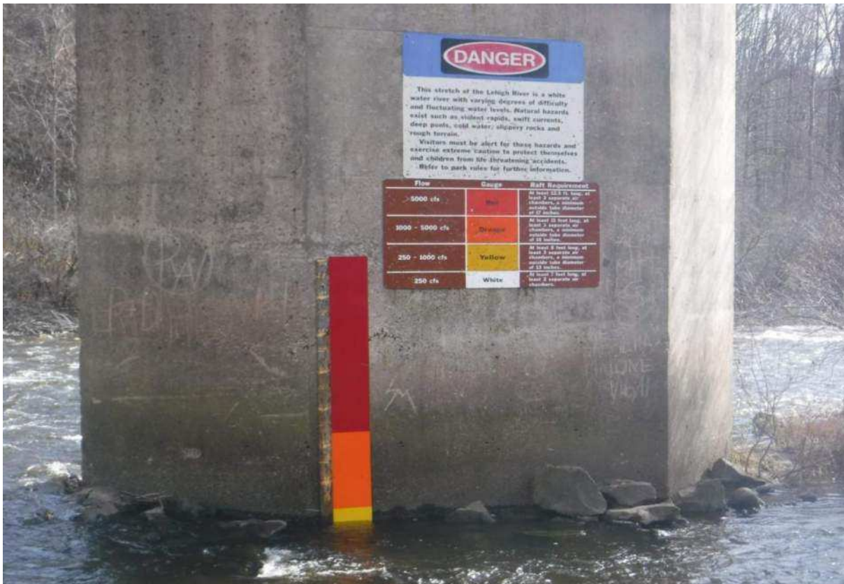
River gauge and raft requirements posted on the eastbound I-80 Lehigh River bridge pier
