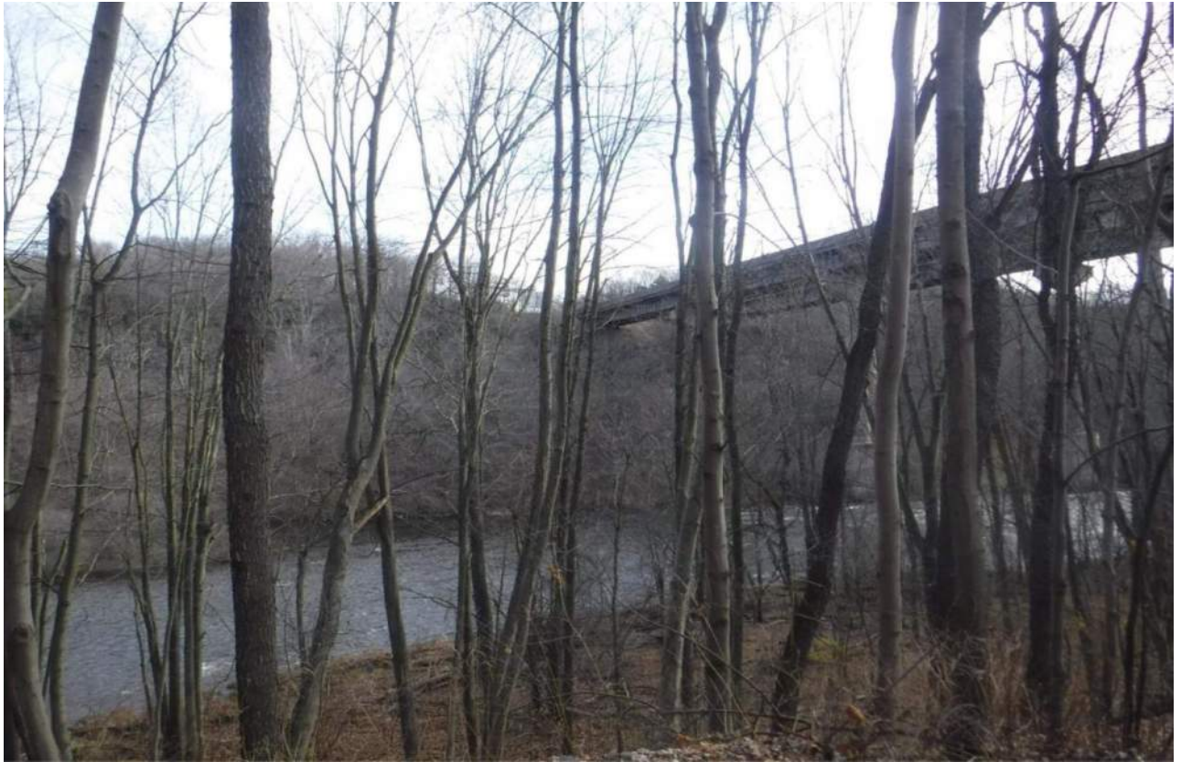
View of I-80 Lehigh River Bridges and Lehigh River, facing southeast
