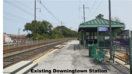
Existing Downingtown Station
