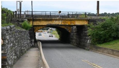
EXISTING BRIDGE - LOOKING SOUTH
