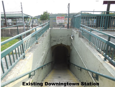
Existing Downingtown Station
