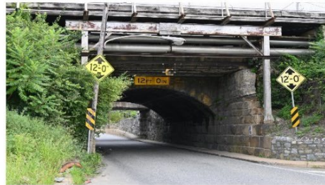
EXISTING BRIDGE - LOOKING NORTH
