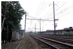
View of the Pennsylvania Railroad Mainline (Philadelphia to Harrisburg and Philadelphia & Columbia Railroad), which share the same tracks and equipment within the project area.
