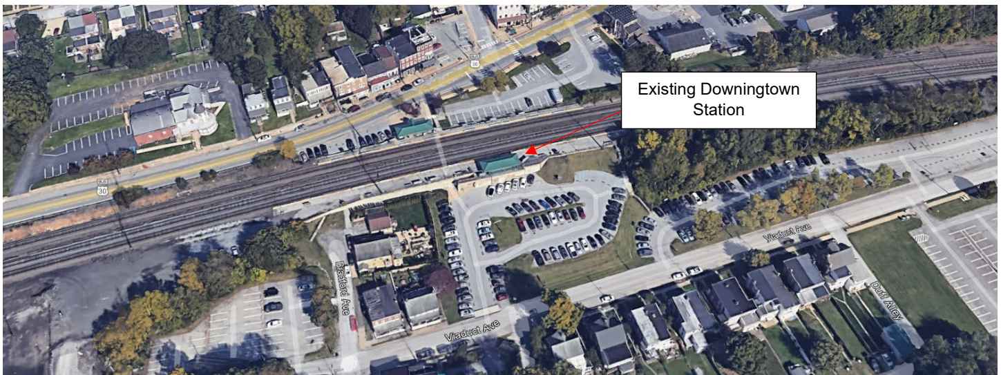
Figure 1: Google Aerial Imagery of Existing Downingtown Station
