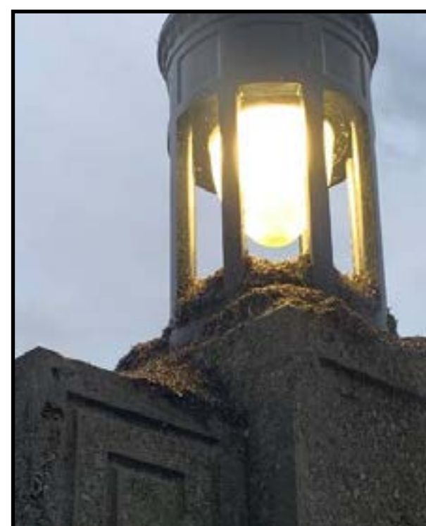
Mayfly deposits at the base of light after one night - existing fixtures
