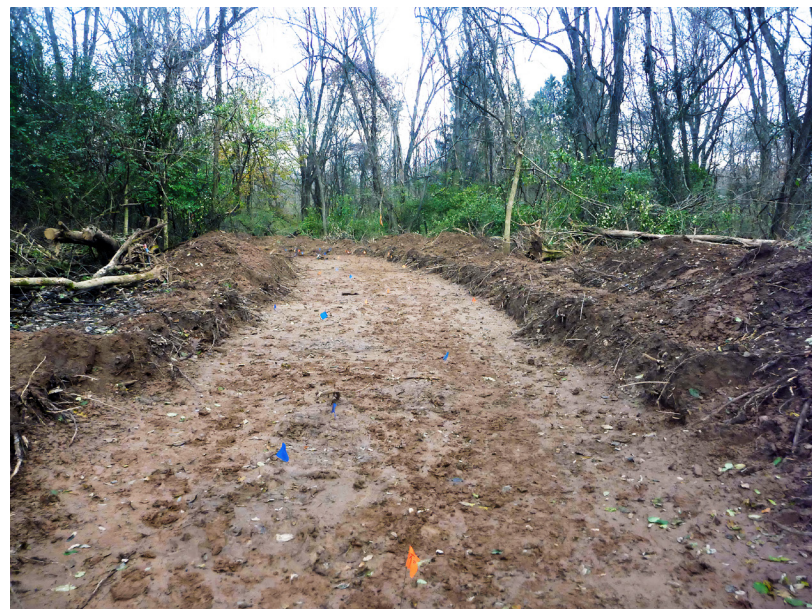
The results of mechanical stripping in a section of SRT-3, November 2018.
