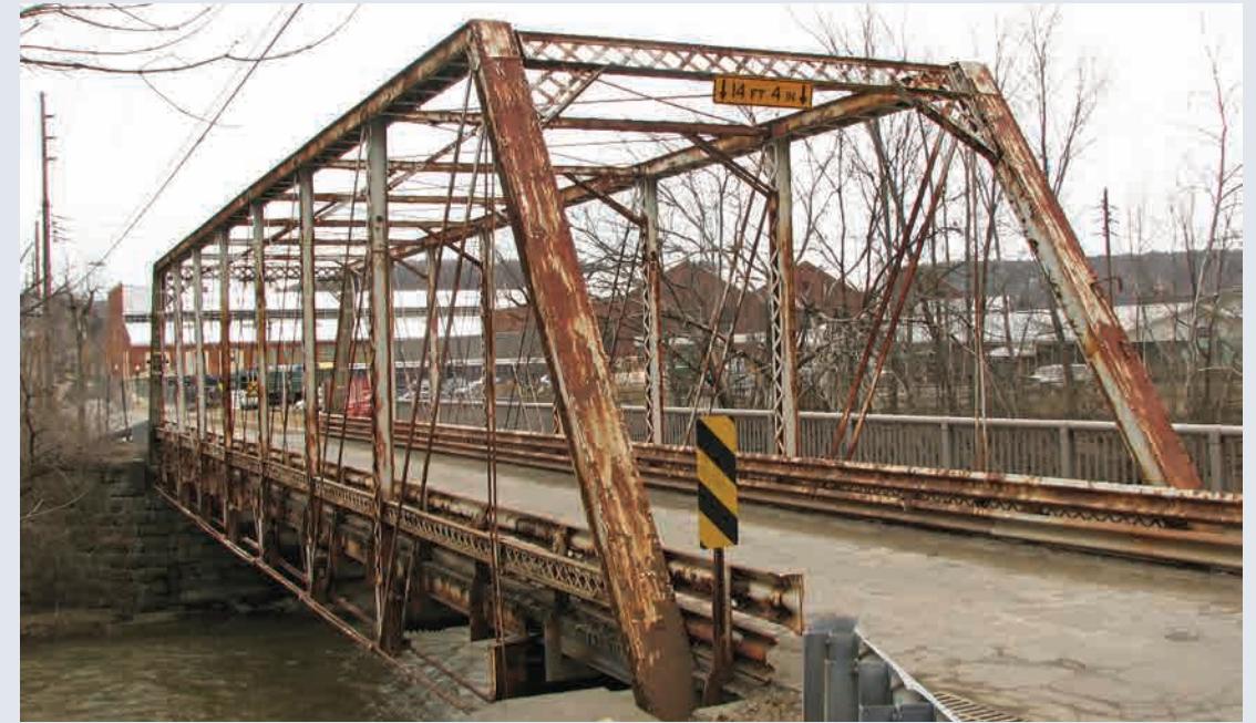
9. South Perry Street Bridge (BUILT 1892)
