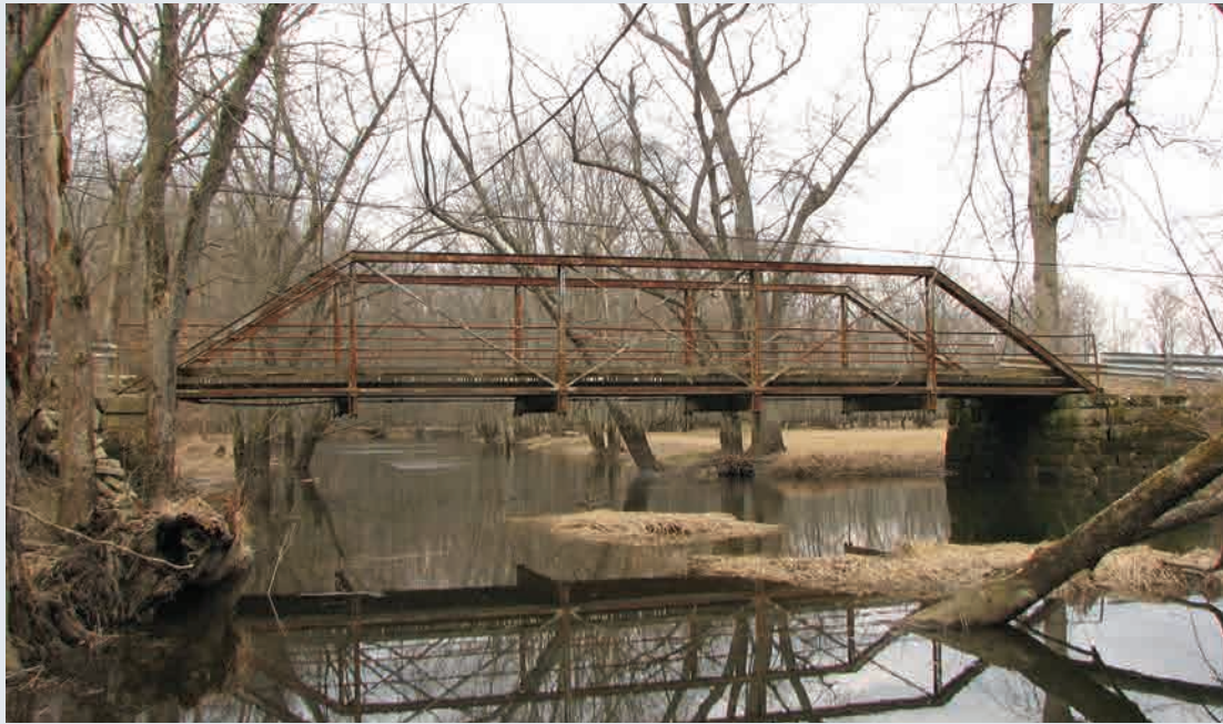
8. Marsh Road Bridge (BUILT 1890)
