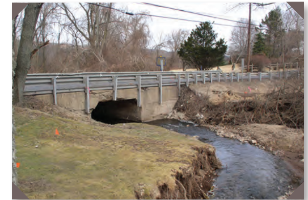
Hellertown Road Bridge over Cook Run.
