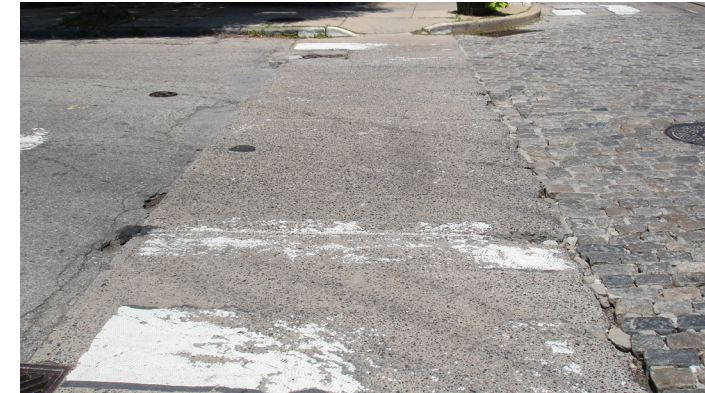
Highland Avenue — observed
