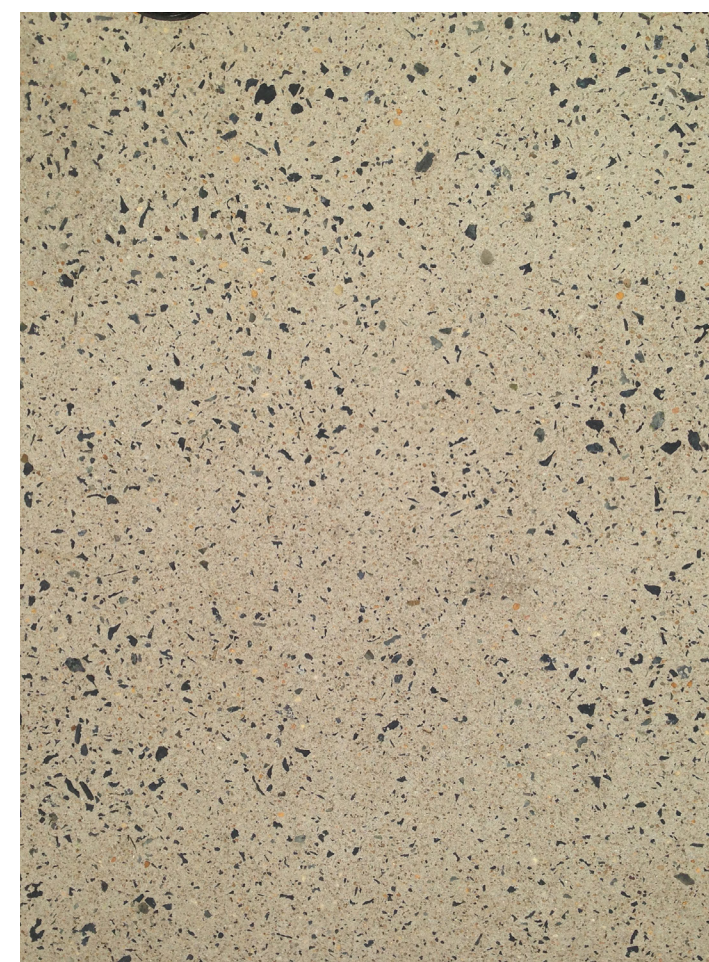
Recommended concrete as seen at Top of the Hill Park
