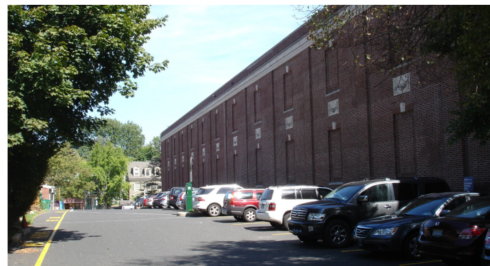
8300 Block Germantown Avenue West Side Orange Lot (Parking Foundation)
