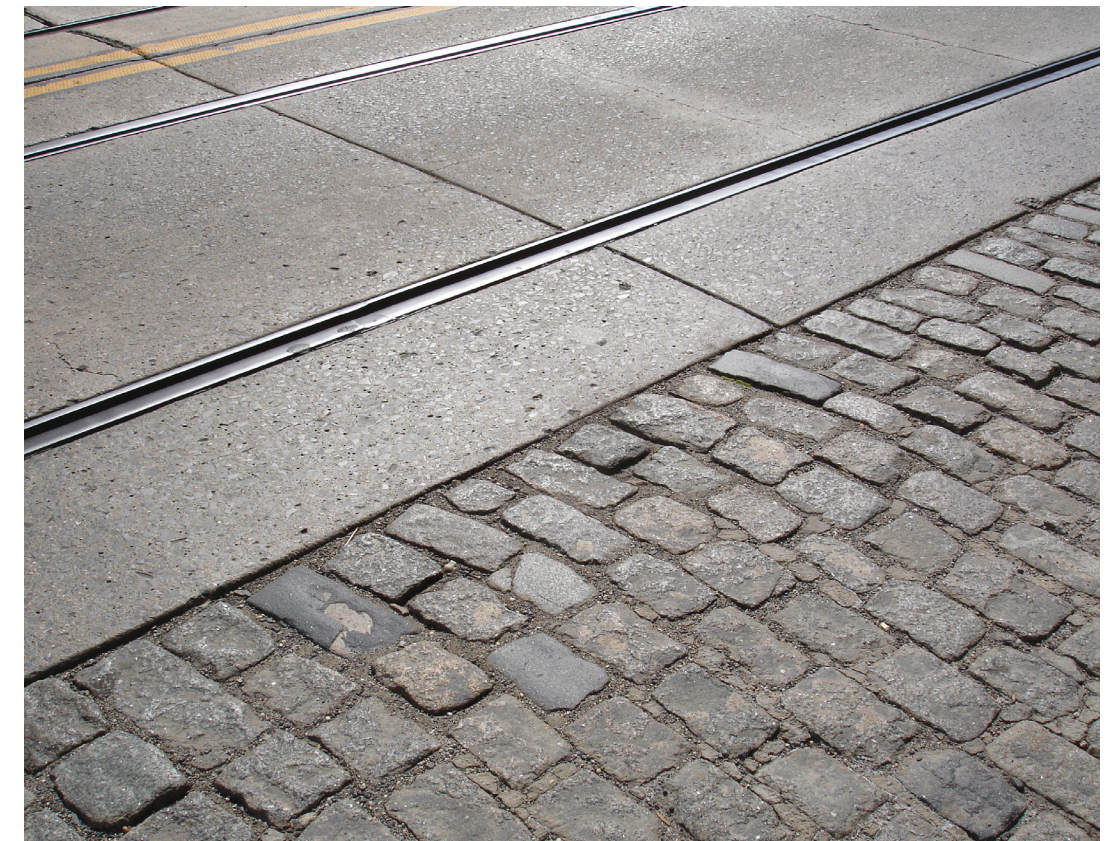
Cobbles, concrete, and trolley tracks in good repair
