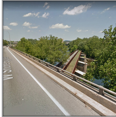
Existing pedestrian bridge (former RR bridge) beneath West Shore Bypass.
