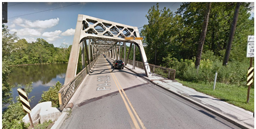
Existing Cementon Bridge
