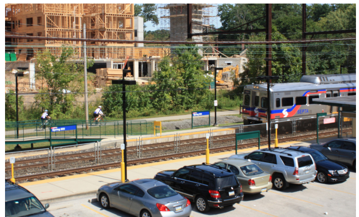
Transit-oriented development is built in Spring Mill, Montgomery County, PA. Photo credit: Montgomery County Planning Commission.
