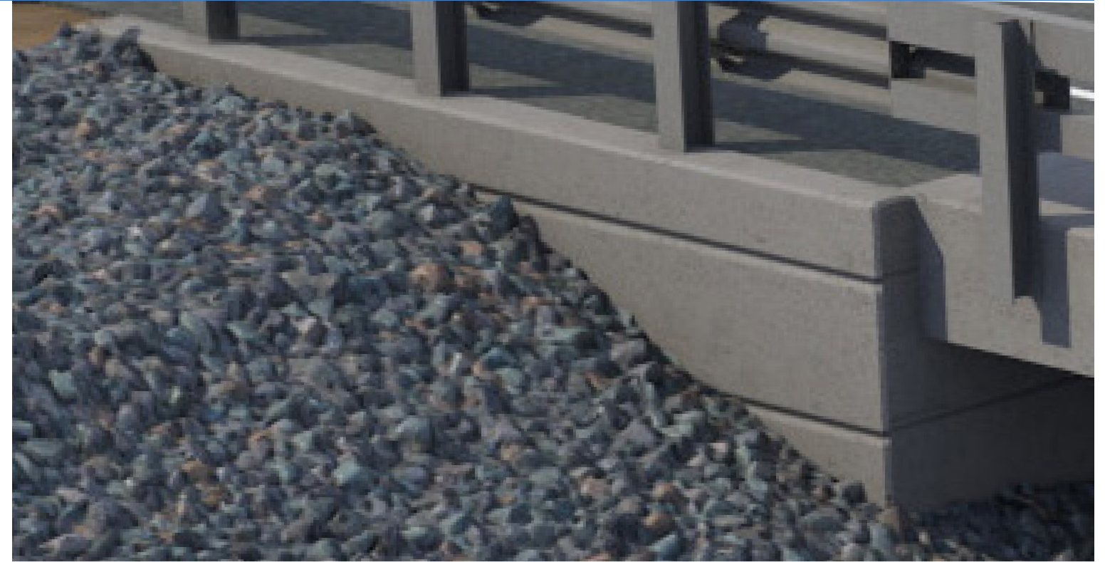
Upgraded wing wall and abutment finish - joint pattern
