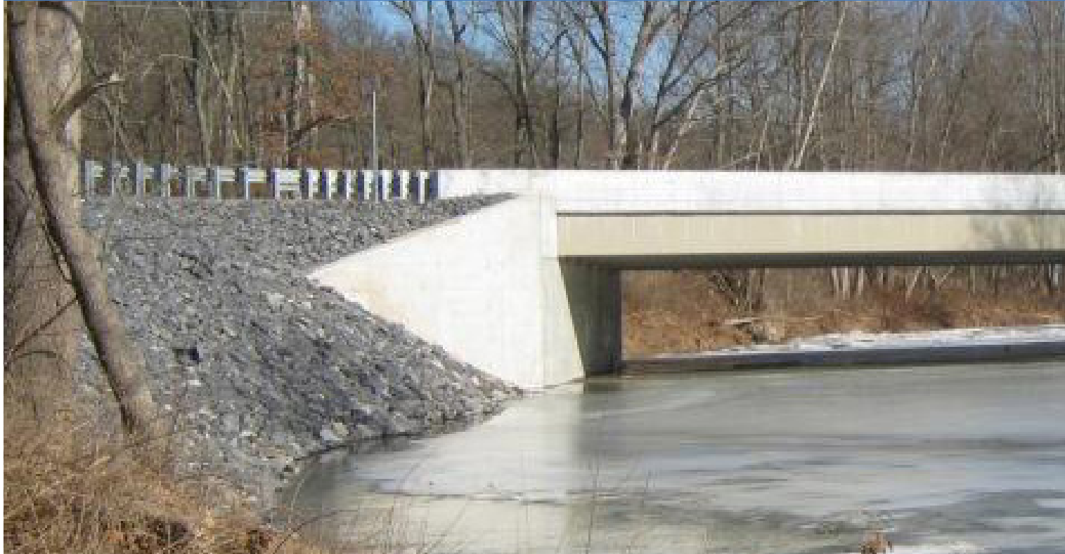
Typical wing wall and abutment finish
