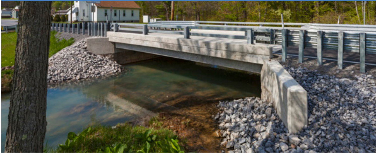
Gravel slope at wing walls
