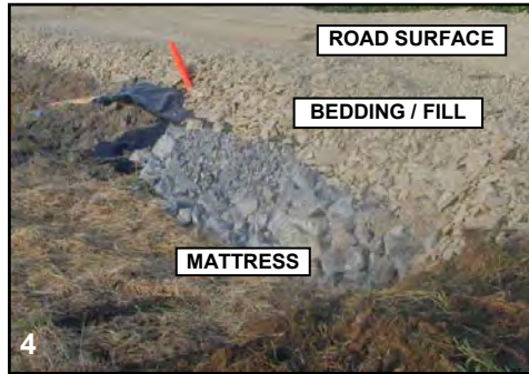
Figures 1-4. French mattress construction sequence.
