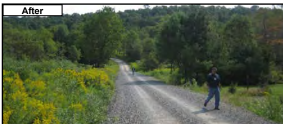
Photo 4. This roadway cuts across a floodplain wetland. A 300 foot long French mattress was used to provide relief for wetland flows while providing a stable road base and preventing beavers from damming the nearby stream pipe.
