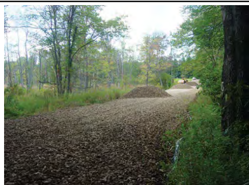
Photo 3. Large mattresses allow wetland flow.
